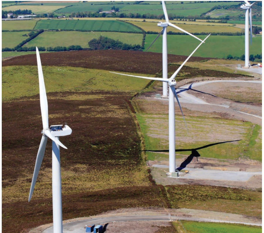
By the end of 2012, ESB had an installed capacity of 334MW of wind farms.
