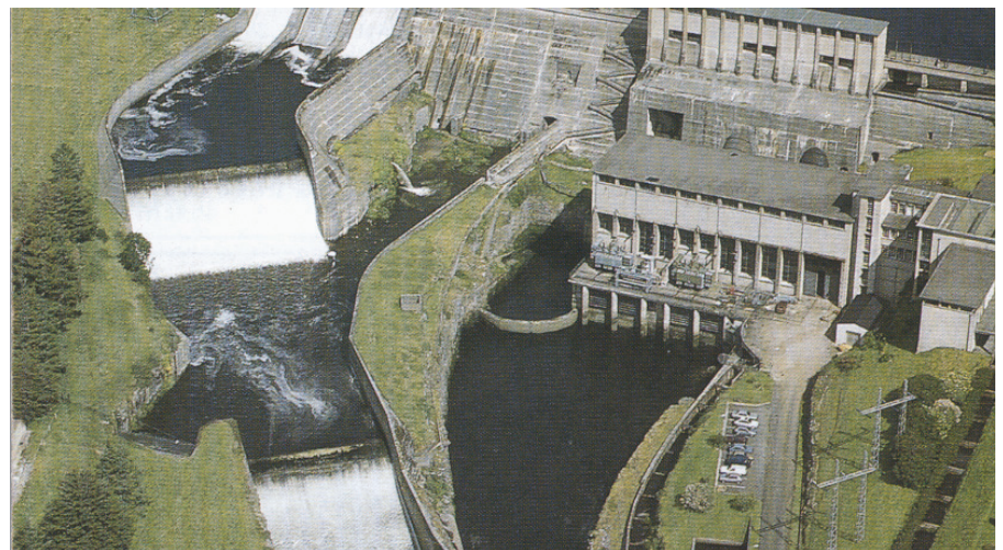
Cathleen's Falls hydro station, Co. Donegal. ESB operates 217MW of hydro and 292MW of pumped storage generation capacity.
