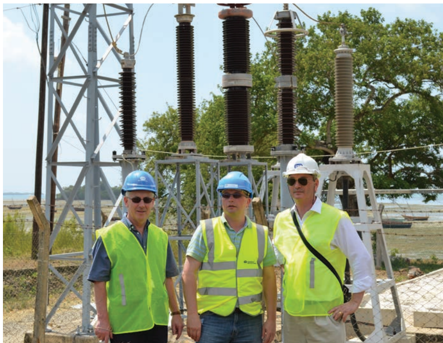
ESB International staff view works completed as part of the Millennium Project in Tanzania.
