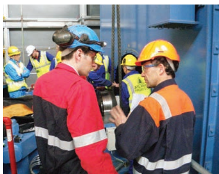
Contractor activity peaks during periods of station overhauls.
