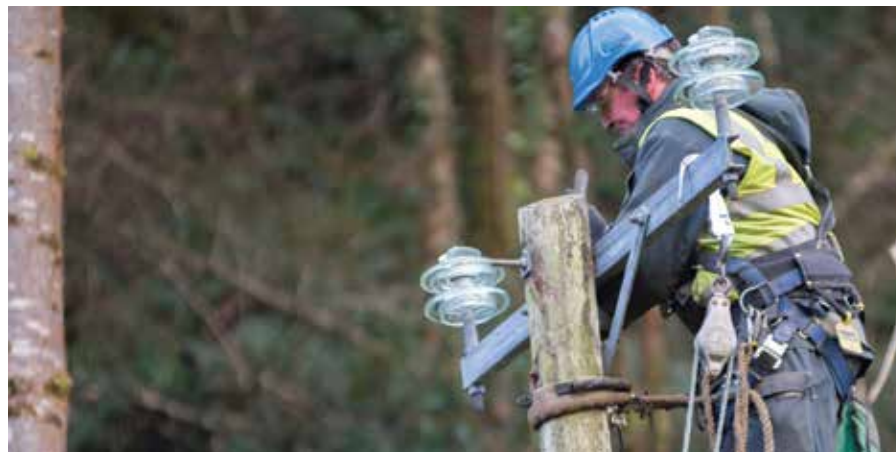
Network Technician working hard to restore power following storm damage
