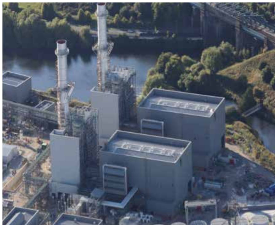
Carrington Power Station, 881MW gas-fired CCGT
