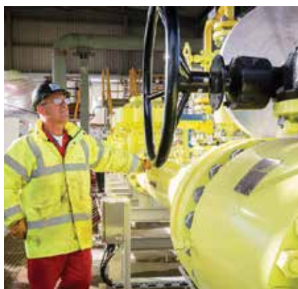
Partnering with contractor organisations is a critical element of constructing large scale assets
