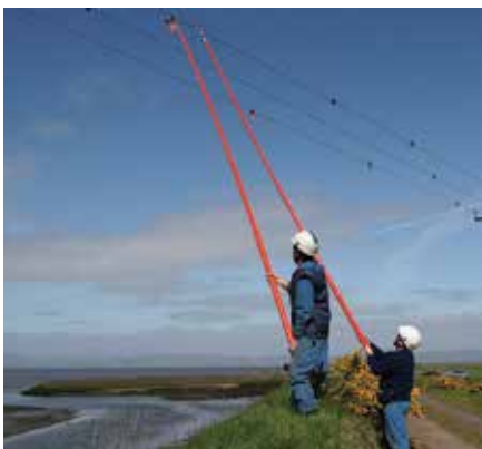
NIE Networks' lines team installing bird diverters
