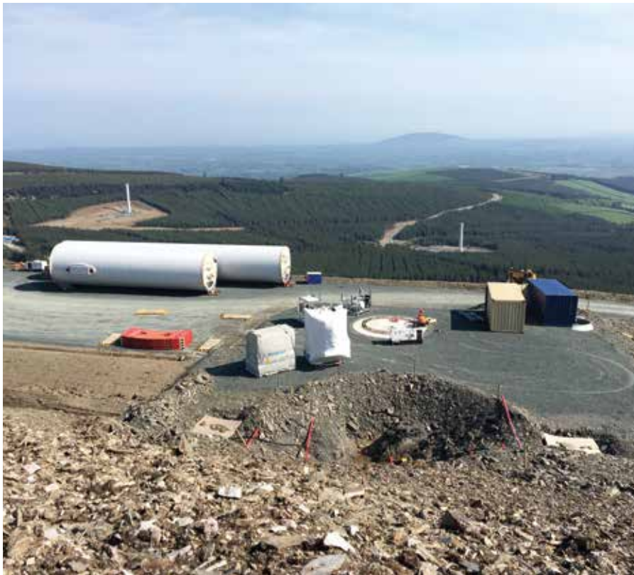
Raheenleagh wind farm under construction
