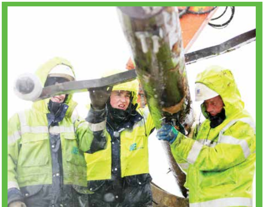
NIE engineers repair damage to the electricity network
