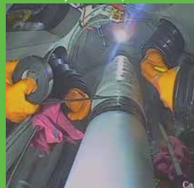
Divers work on the repair inside the submersible habitat
