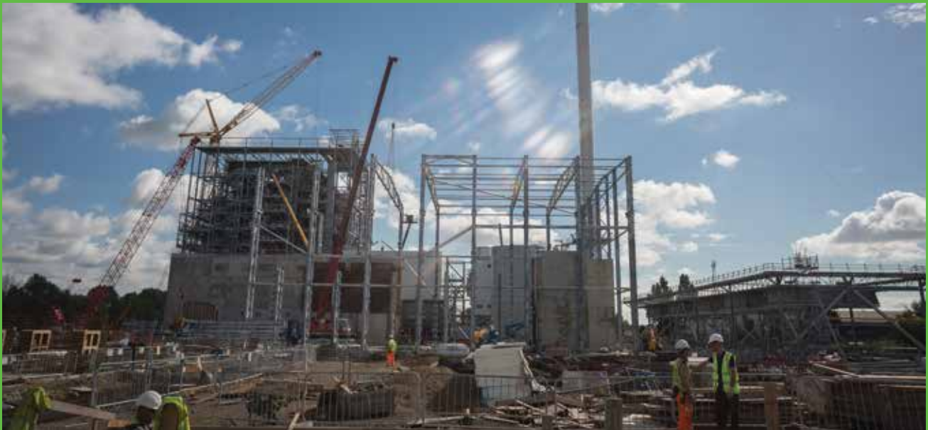
Tilbury 40MW Biomass site in London, UK, under construction
