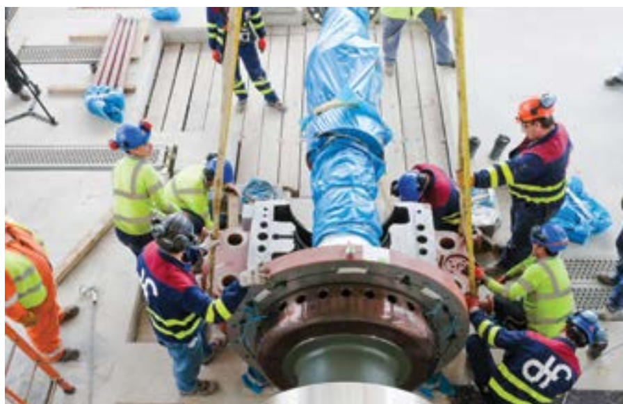
Turbine shaft installation in Carrington 881MW CCGT.
