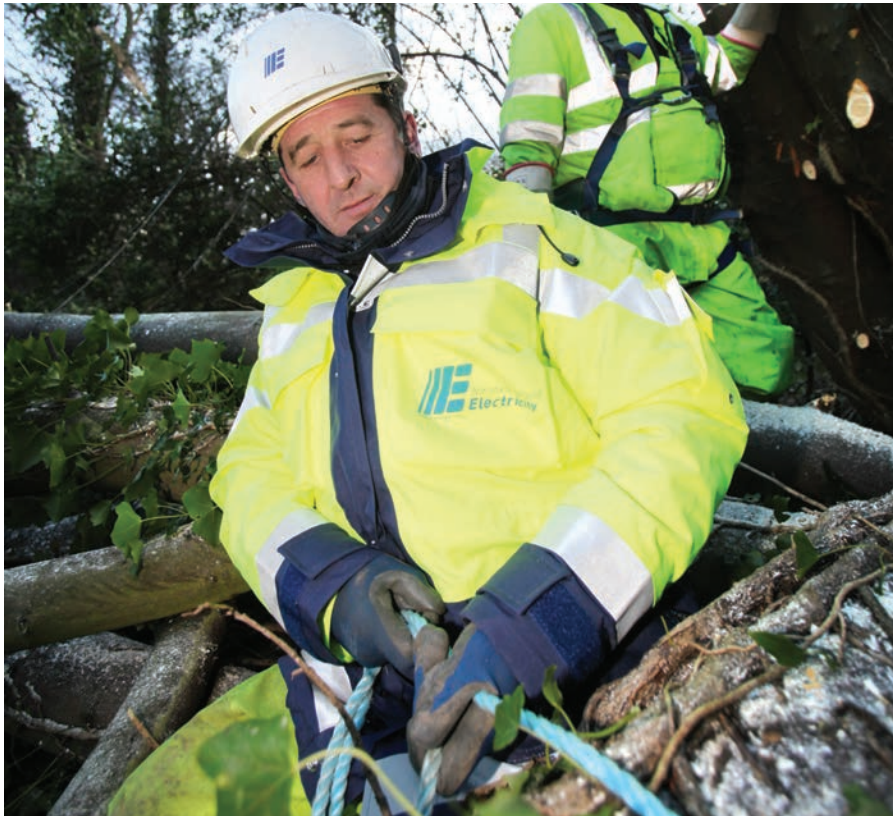
NIE Crew work to restore supply following a storm.
