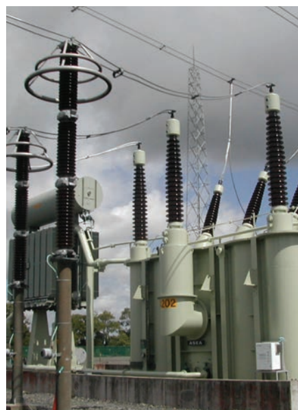
SF6 gas is widely used in transformer cooling.
