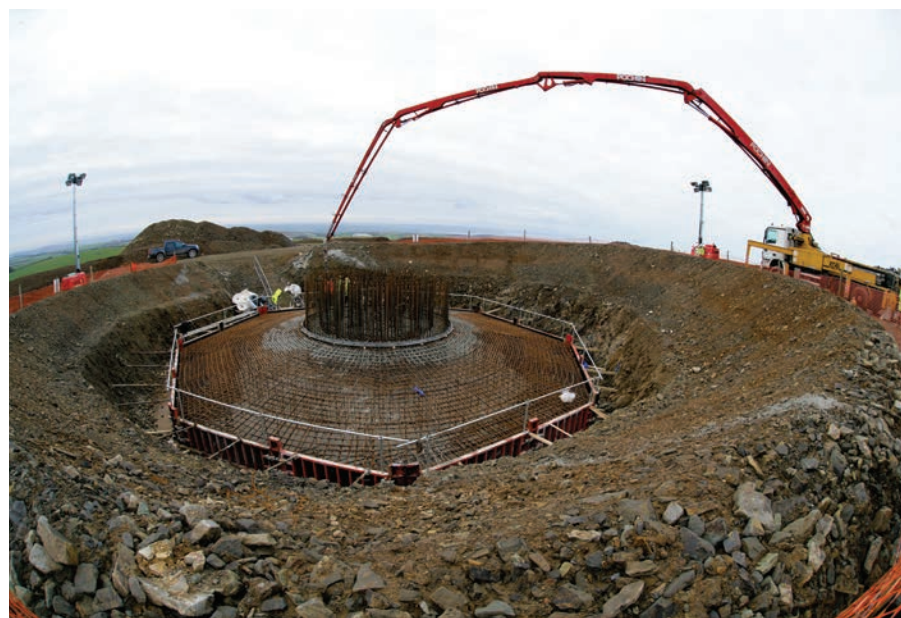
ESB uses 75% environmentally-friendly cement (Ecocem) in our wind turbine foundation mixes.
