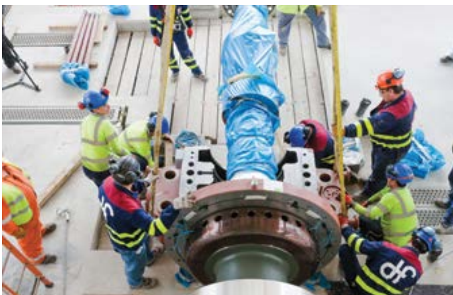
Turbine shaft installation in Carrington 881MW CCGT.
