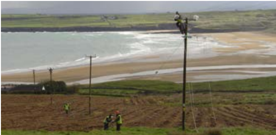
Preparation works for a 20kV conversion of an MV network.
