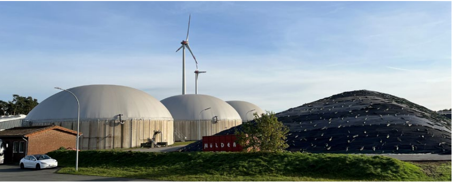
An anaerobic digester in Germany
