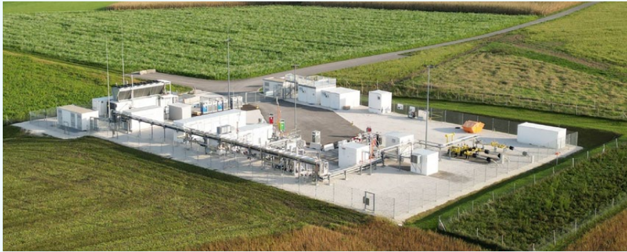
Underground hydrogen storage in Austria (Credit: RAG Austria)
