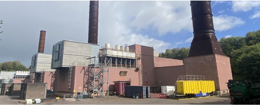
HVO fuel trials at ESB's Aghada Power Station
