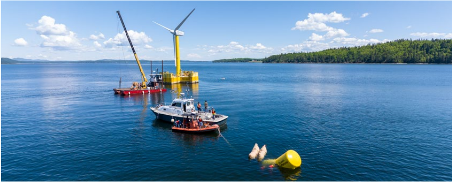
Dublin Offshore Technology's Load Reduction Device being installed in the Gulf of Maine in the US. The operation was part of a demonstration of the DeepCwind VoltturnUS+ concrete floating wind turbine foundation (Credit: Dublin Offshore Technology)
