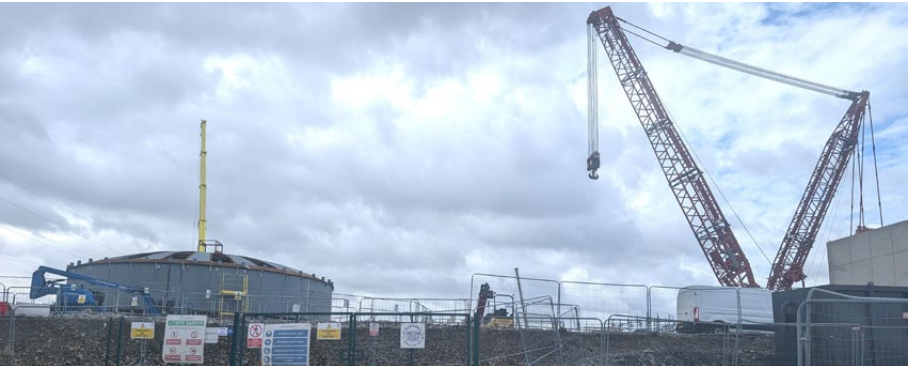
Highview Power's Liquid Air Energy Storage plant under construction near Manchester, UK
