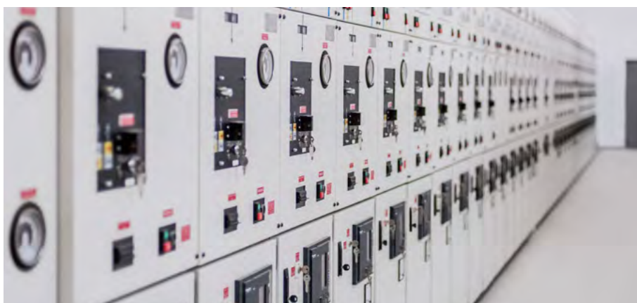
Metal enclosed switchgear
