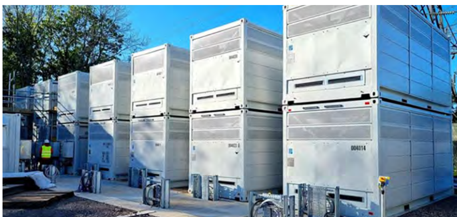
Vanadium Flow Batteries in Oxford, UK (Credit: Invinity)
