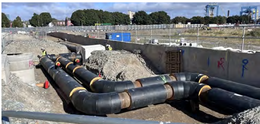
DDH pipes (Credit: RTE)
