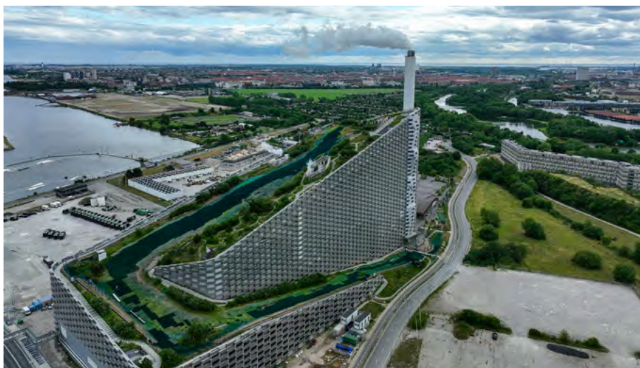
Amager Bakke waste-to-energy plant in Copenhagen includes carbon capture.
