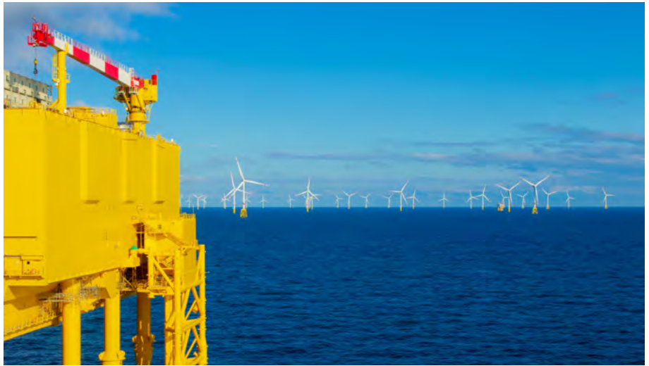
North Sea Offshore HVDC Substation
