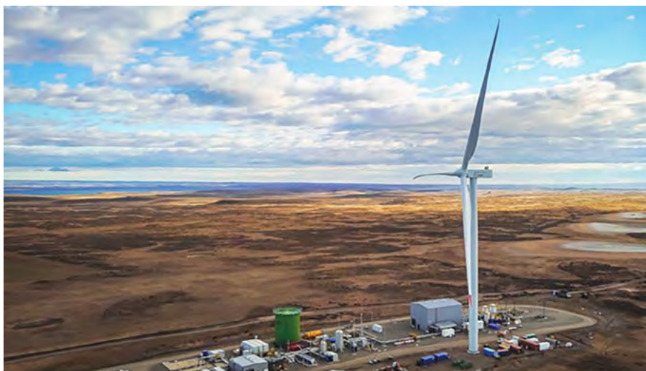
'HIF' e-diesel pilot plant, Magallanes, Chile. Credit: HIF
