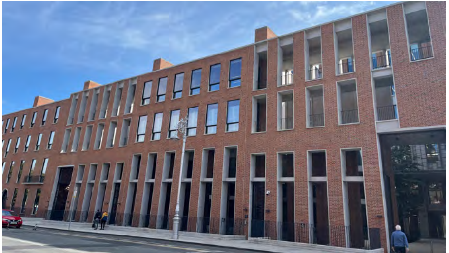
ESB Head Office uses Ground Source Heat Pumps
