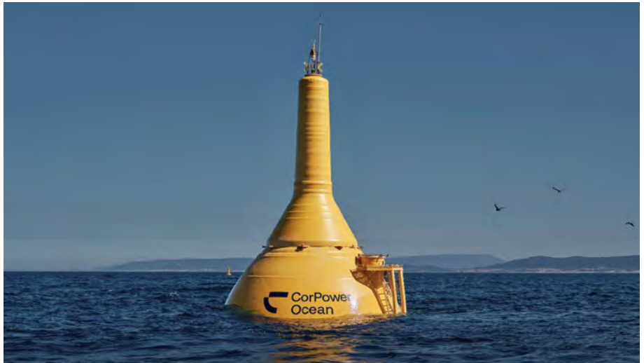
Wave energy converter, deployed in Portugal. Credit: Corpower
