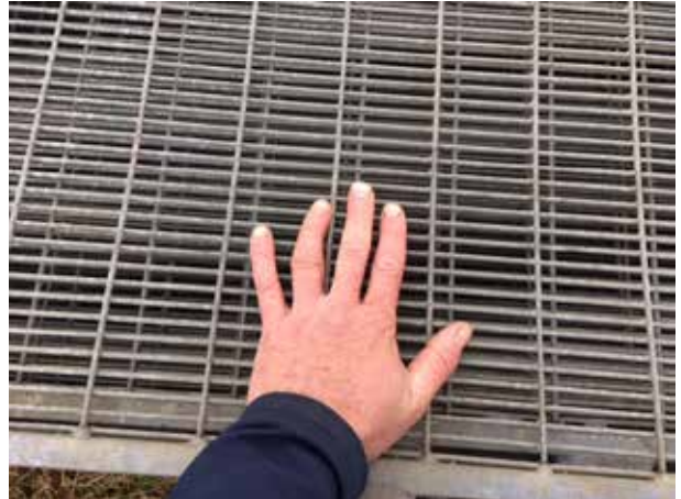
A photograph of the one of the salmon smolt screens which are fitted to the intake canal of Clady station, prior to the annual smolt migration.
