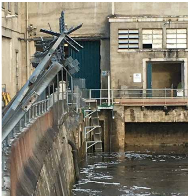
A new elver trap located downstream of Ardnacrusha on the north bank.
