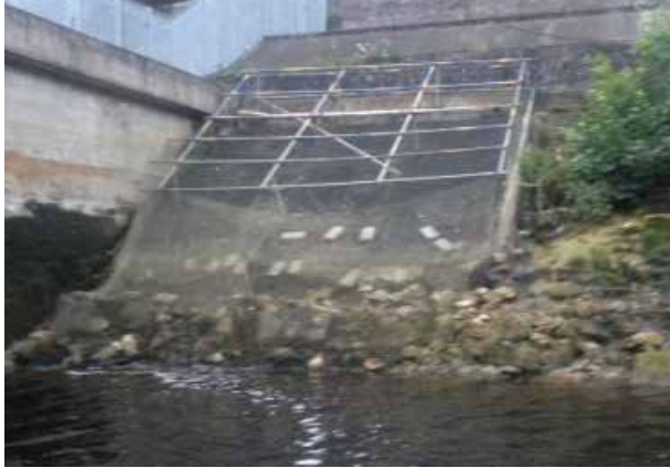
Before and after views of the Ardnacrusha elver trap with the new elver climbing substrate and water supplies added. Also included are a new walkway, attraction flow and diversion of existing flows onto the ramp area. A new elver collection box was also added to facilitate the trapping of elvers from the area in front of the Borland Fish lift.
