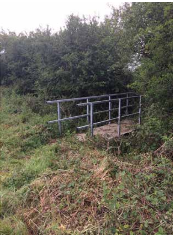
Access improvements on Mulkear river.
