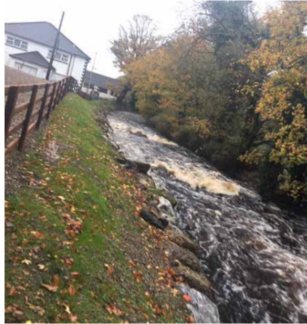
The Woodford River in high flows with a series of instream stone weirs and rock armor along the near side of the riverbank.
