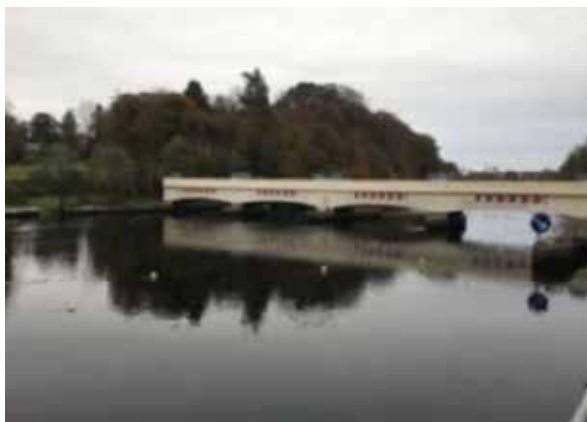
The 'Portora Gates' site on the mid Erne catchment (Enniskillen town).
