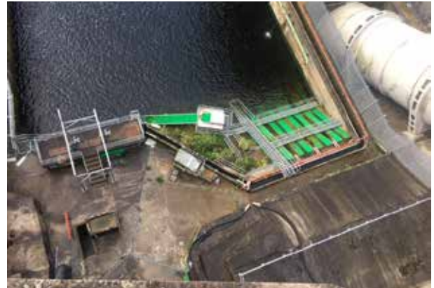
An aerial view of the upgraded Ardnacrusha elver trapping facilities.
