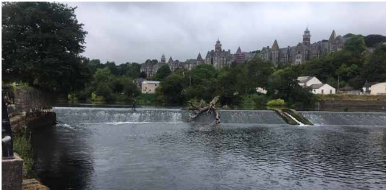
A view of the south side of the Lee Weir showing the centrally located fish pass.
