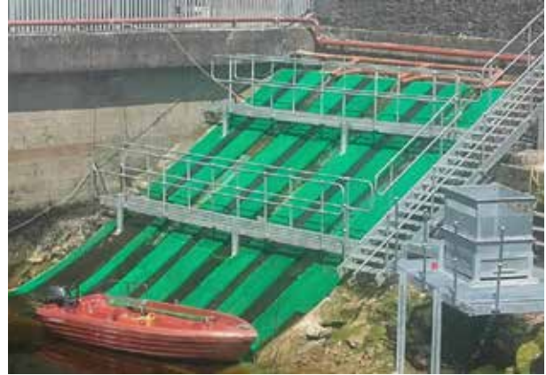
Before and after views of the Ardnacrusha elver trap with the new elver climbing substrate and water supplies added. Also included are a new walkway, attraction flow and diversion of existing flows onto the ramp area. A new elver collection box was also added to facilitate the trapping of elvers from the area in front of the Borland Fish lift.
