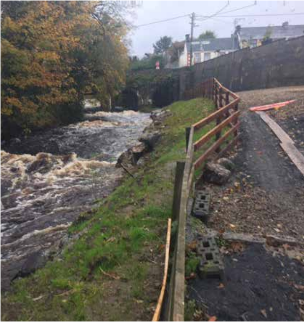
The Woodford River in high flows with a series of instream stone weirs and rock armor along the near side of the riverbank.
