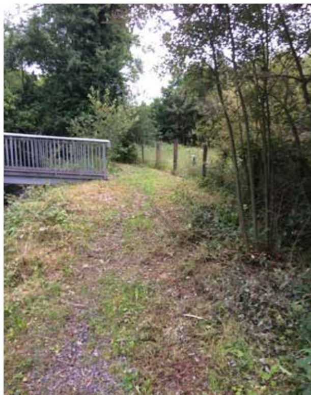
The access path to the footbridge on the Camcor River.
