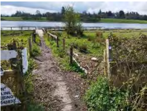
Catwalk access and fencing at Clonahee prior to works.
