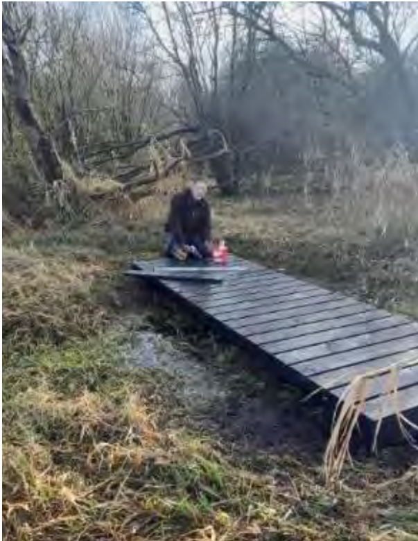
The construction of footbridge on a tributary of the R. Inny at Coolnagun.
