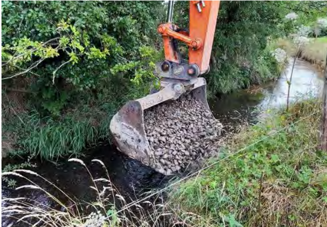
The addition of spawning gravels into the Pound River.
