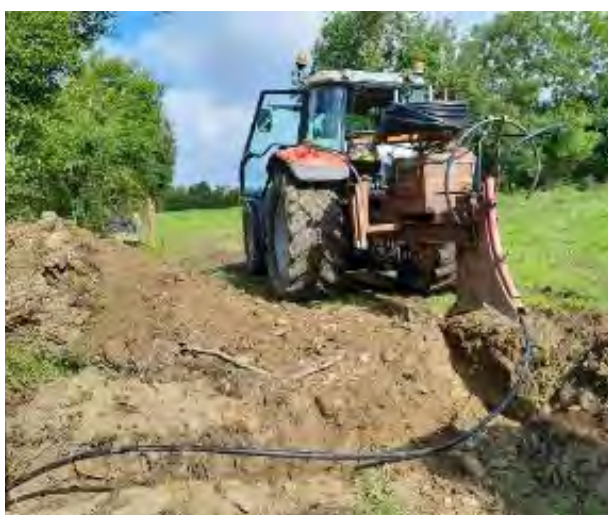
The laying of piping for drinkers (left); and a drinker installation (right) which were undertaken as part of the Mountnugent Instream Enhancement project.
