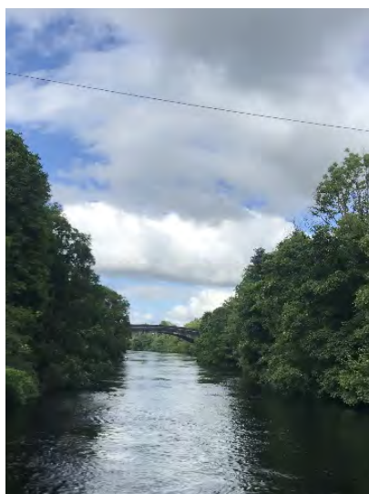
A section of the Ardnacrusha tailrace.
