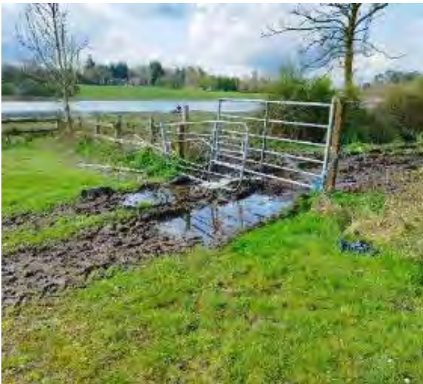
Car-park and fencing at the Clonahee fisher prior to works.
