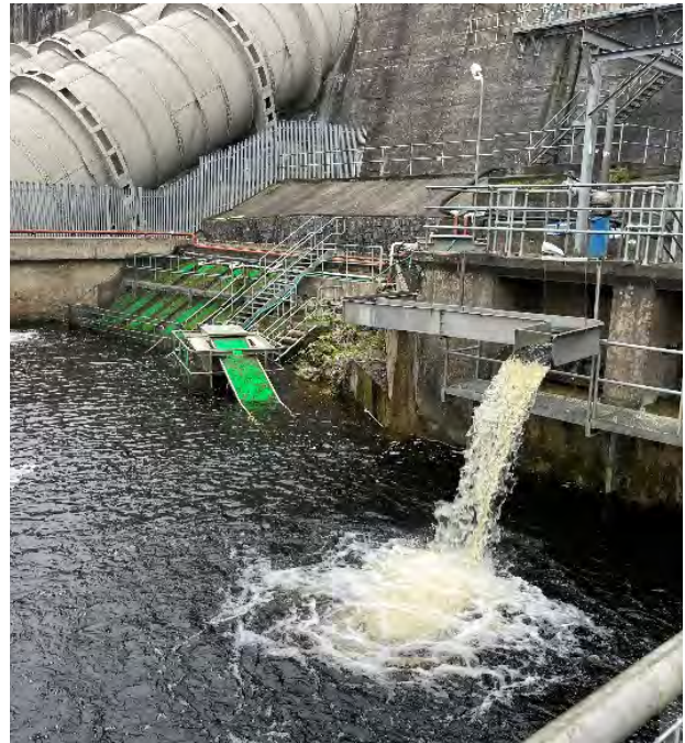
The Ardnacrusha juvenile eel trap with the green coloured climbing substrate and the cooling water being discharged beside the juvenile eel trap ramp. Cooling water from the station is also discharged at the entrance to the Ardnacrusha fish lift as a fish attraction flow.
