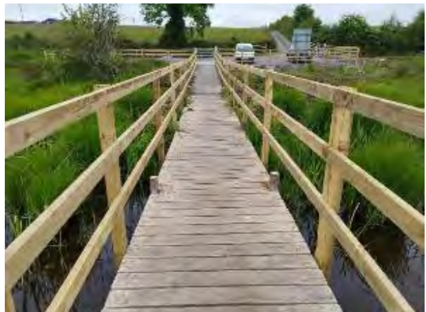
Catwalk access and fencing at Clonahee post work.
