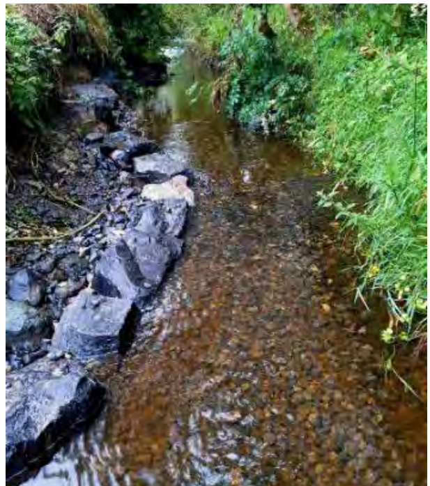
An instream deflector and spawning gravels on the Finaway River.
