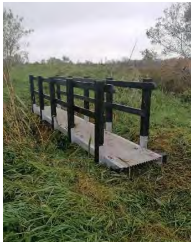
A pre-made 17ft bridge ready for placement at Camagh on the River Inny.
