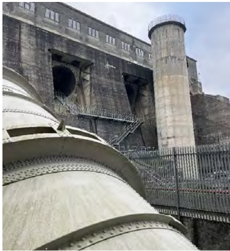
A view of one of the Ardnacrusha penstock pipes and the Ardnacrusha Borland Fish lock behind.
