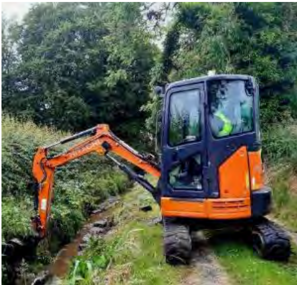
The construction of alternating deflectors on the Maghera River (left) and the addition of spawning gravels (right).
