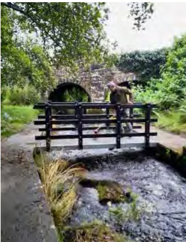
A new footbridge at Creggs Village, Co Galway (Suck catchment).
