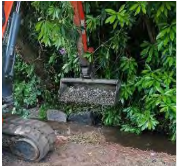
The construction of alternating deflectors on the Maghera River (left) and the addition of spawning gravels (right).
