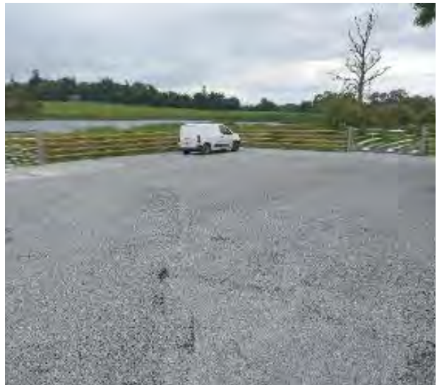
Car-park and fencing at the Clonahee fisher post works.
