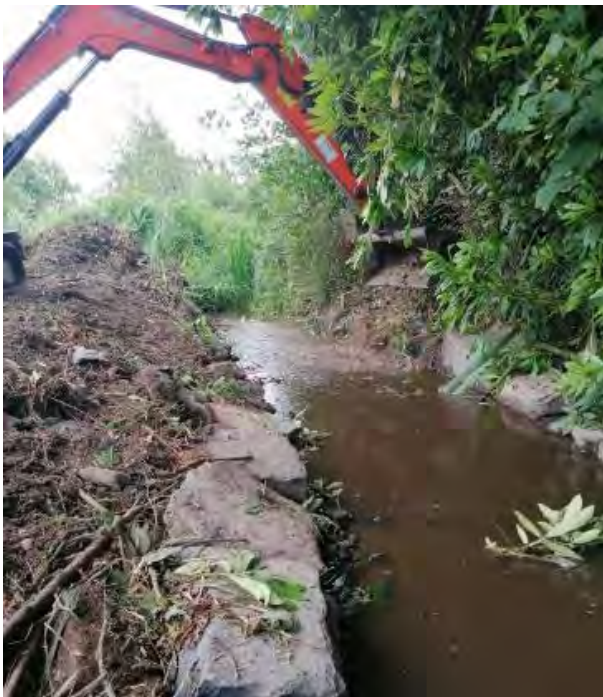
Bank protection and spawning gravels being added to the Finaway River.
