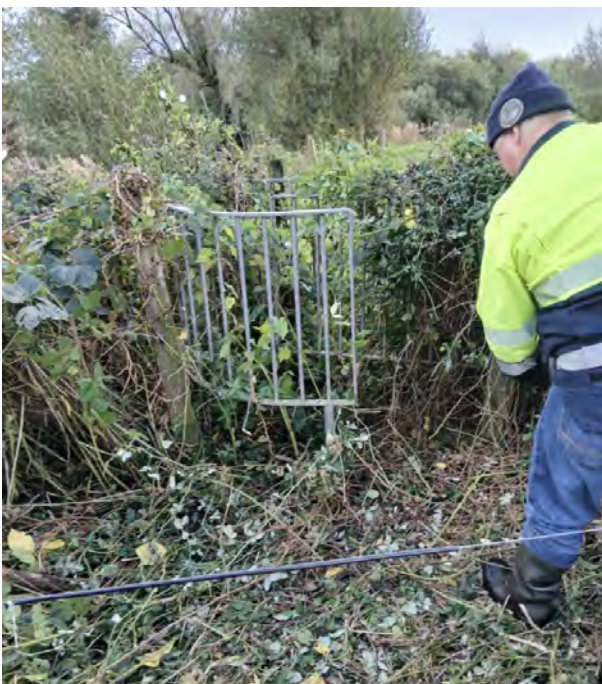
Clearing footpaths and swing gates at access points on the banks of the Mulkear fishery.
