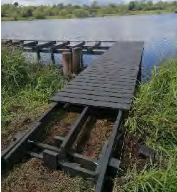
The construction of a double fishing stand at Fearglass, Longford.
