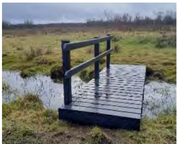
A new footbridge constructed along the main River Inny.
