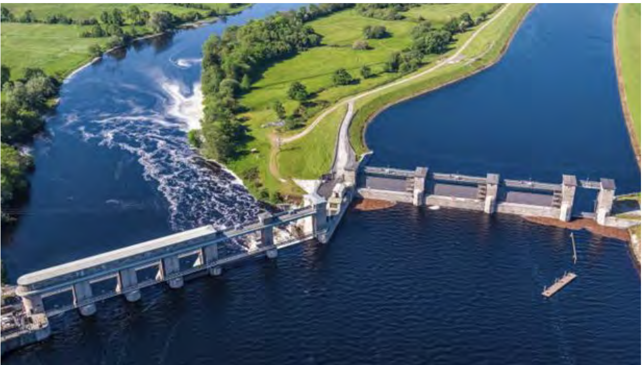
An aerial photograph of Parteen Regulating weir on the Old River Shannon and the Ardnacrusha intake gates on the headrace canal.
