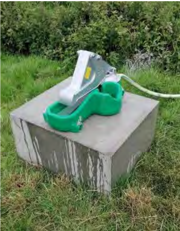
The installation of 'nose' pumps for livestock, which are placed 30m back from Maghera River.
