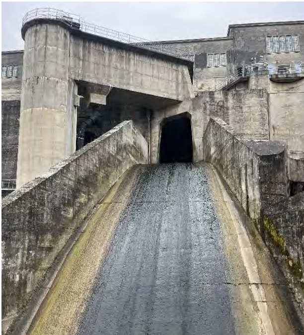
A view of the downstream section of the Ardnacrusha spillway.
