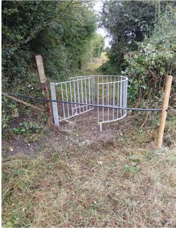
A pedestrian gate recently erected at Riverstown section of the Little Brosna in 2024.
