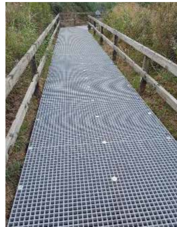
New GRP surface on the existing all-access angling stands at Donamon.
