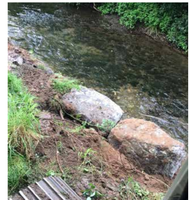
A short section of rack armour being built on the Ballyfinboy River.
