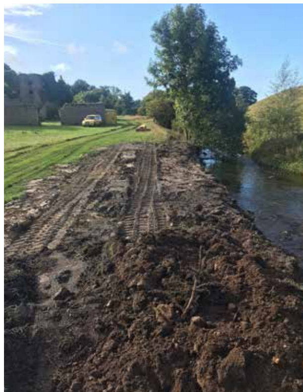
Ground being levelled and the refilling of the riverbank after the placement of bankside rock armour.
