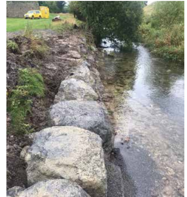
A short section of rack armour being built on the Ballyfinboy River.
