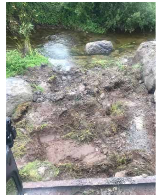
A random boulder being placed into the Ballyfinboy River.
