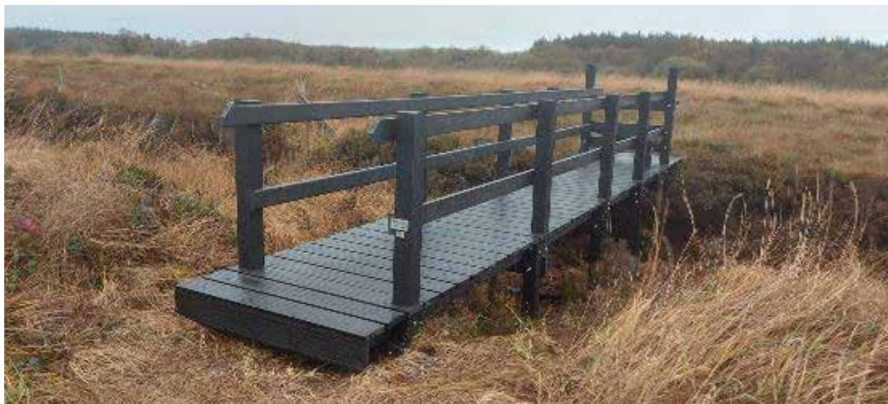
New footbridge access at the River Lung, near Lough Gara.
