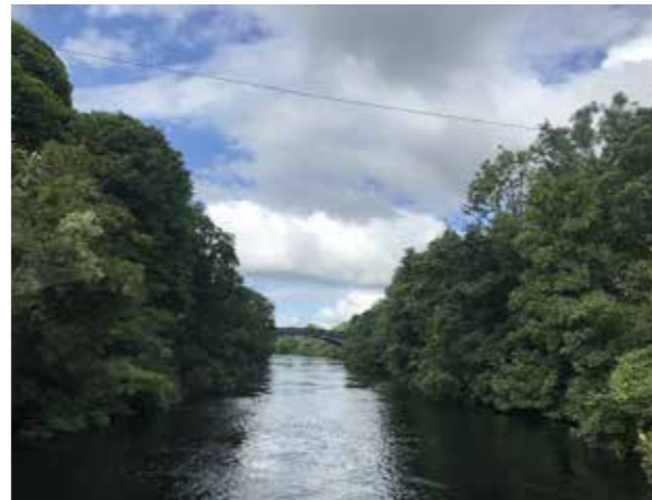
A section of the Ardnacrusha tailrace.
