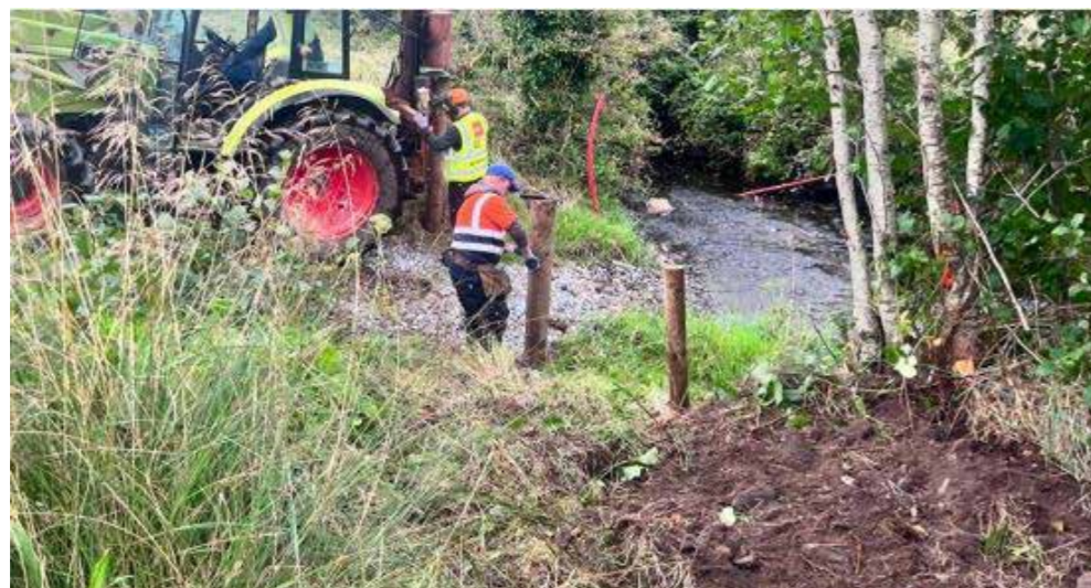
Fencing and solar pump installation at Ballindrumlea (Francis River).
