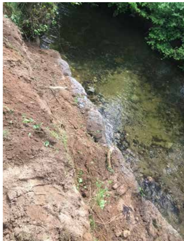
Ground being levelled and the refilling of the riverbank after the placement of bankside rock armour.
