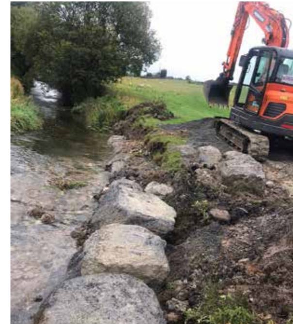
A short section of rack armour being built on the Ballyfinboy River.
