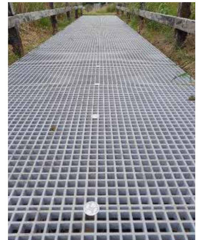
New GRP surface on the existing all-access angling stands at Donamon.
