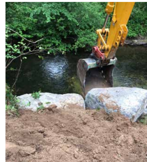
A short section of rack armour being built on the Ballyfinboy River.
