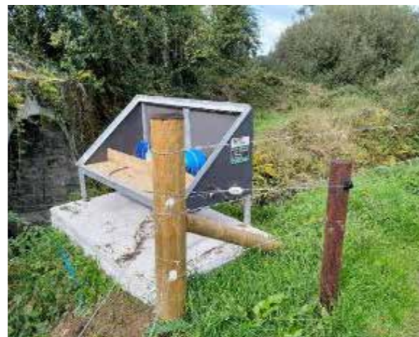
Solar pump on a precast concrete base and the pump insertion on the Pound River.
