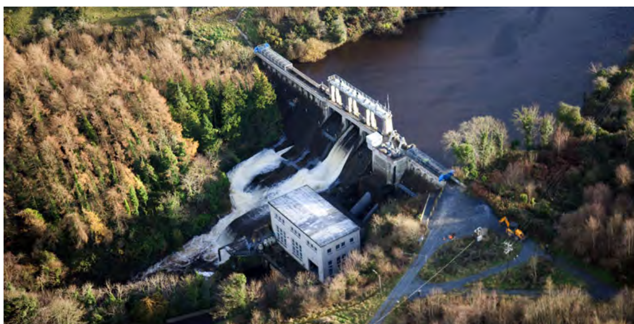
Carrigadrohid Hydropower Station.
