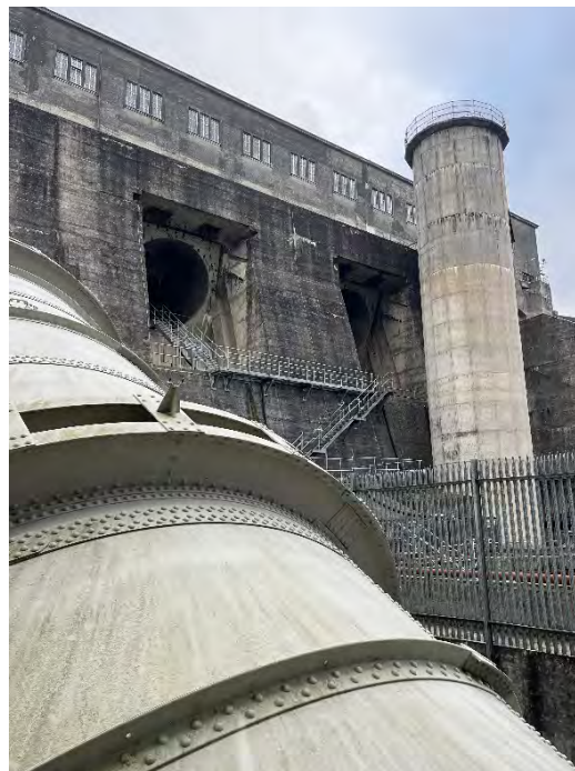
A view of one of the Ardnacrusha penstock pipes and the Ardnacrusha Borland Fish lock behind.
