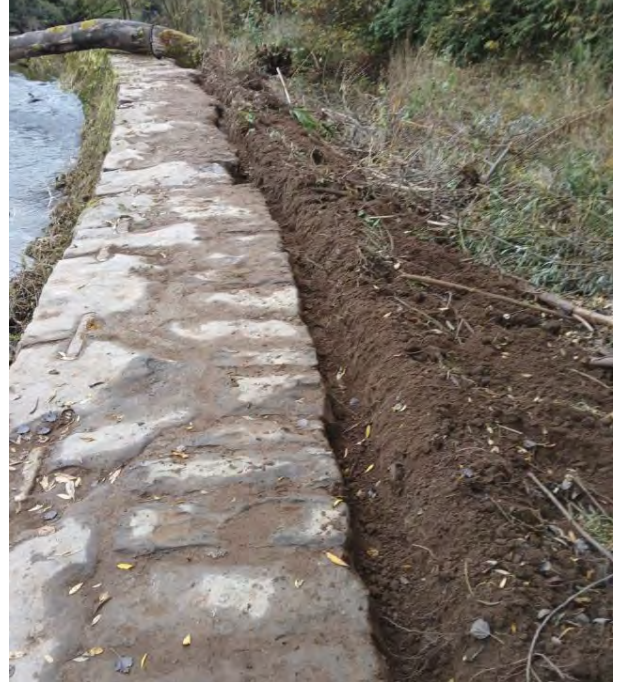
Ballyclough Weir on the Mulkear River, being cleared to allow access onto the weir wall.
