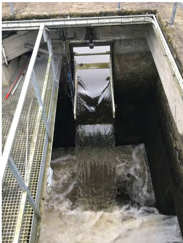
Water spilling into the upper entry point of the Leixlip station Borland fish lock, during the 2023 salmon smolt and elver generation protocol.
