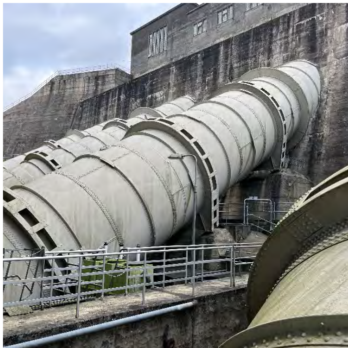
A view of the four Ardnacrusha penstocks which take water from the headrace canal to the turbine units.
