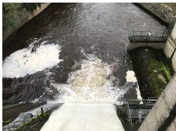
Water spillage through the 'trash flap' gate at Leixlip station as part of the 2024 smolt generation protocol.
