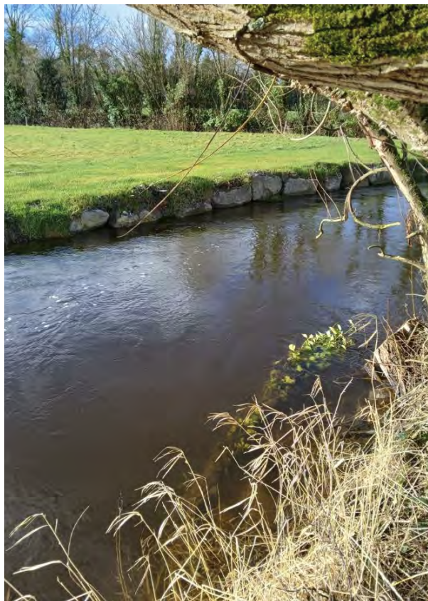
A length of riverbank where rock armoring of the bankside has been completed.
