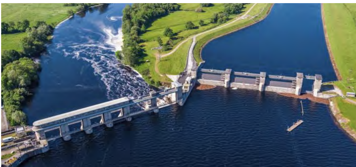
An aerial photograph of Parteen Regulating weir on the Old River Shannon and the Ardnacrusha intake gates on the headrace canal.
