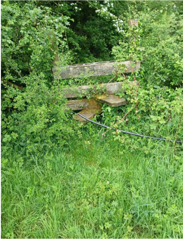
A wooden stile which will be replaced with a pedestrian gate.
