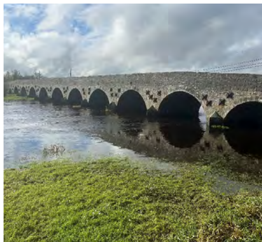
A bridge over the River Suck at Abbeyshrule.
