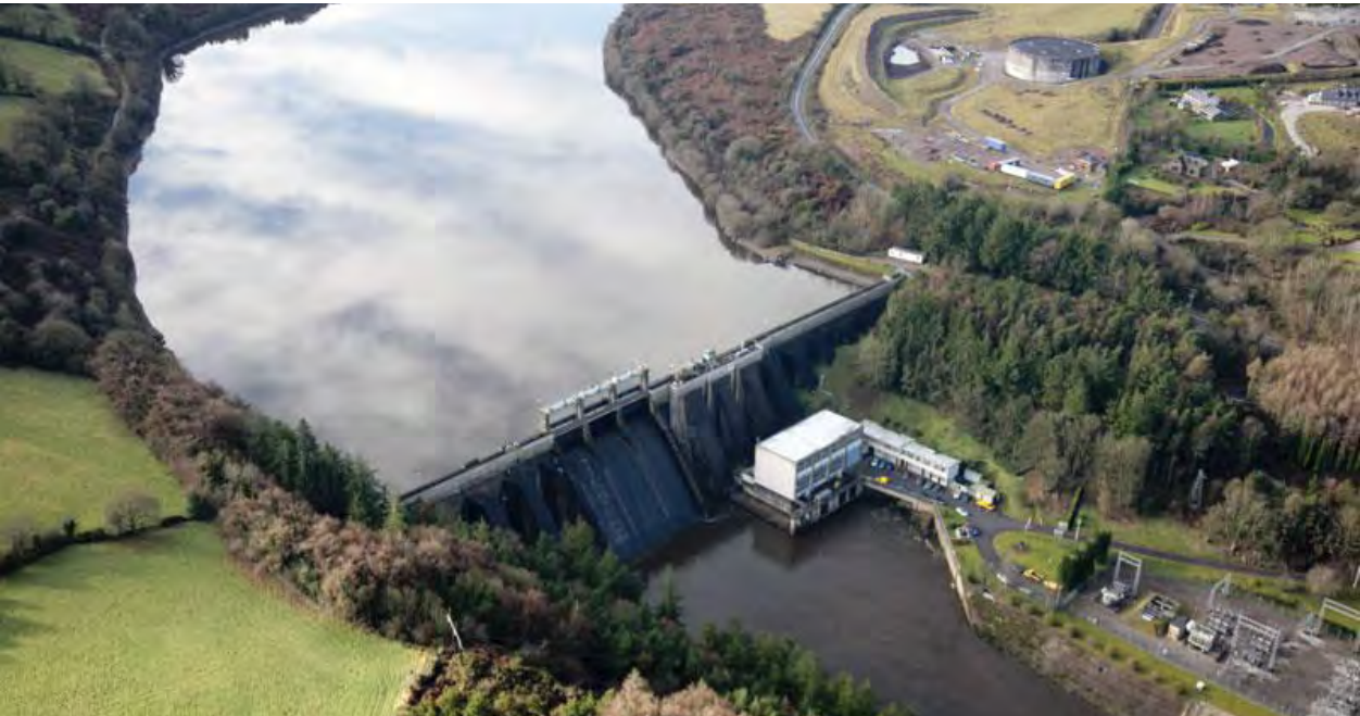
Iniscarra Hydropower Station.
