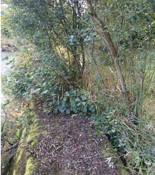
Ballyclough Weir on the Mulkear River, prior to work commencing.
