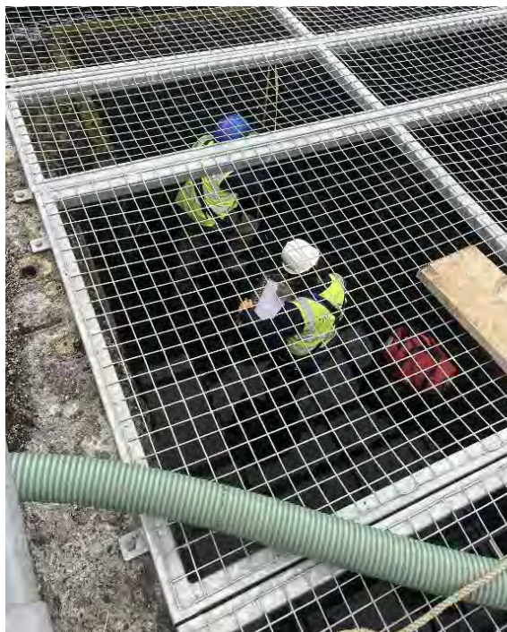
Fish passage consultants undertaking an assessment of the Cathleen's Fall fish pass.
