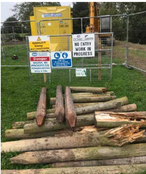
ESB Fisheries safety signage and both new and old fencing posts being used for site fencing in 2023.
