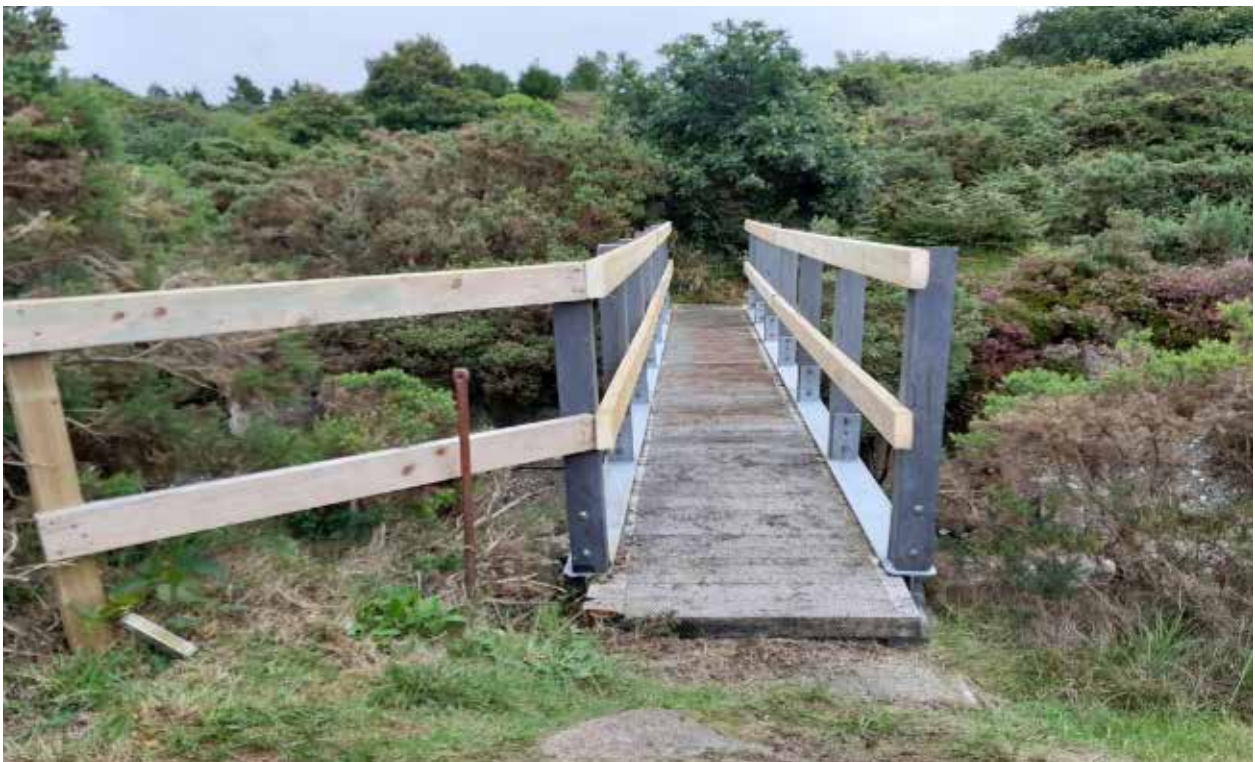
New repairs to the Clady River footbridge.
