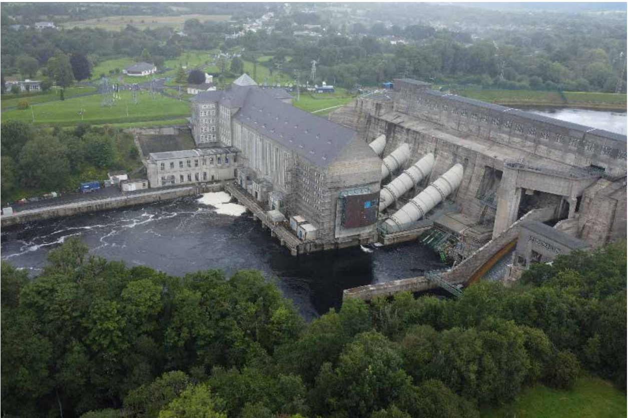
IFI drone footage showing Ardnacrusha station on the Lower Shannon.
