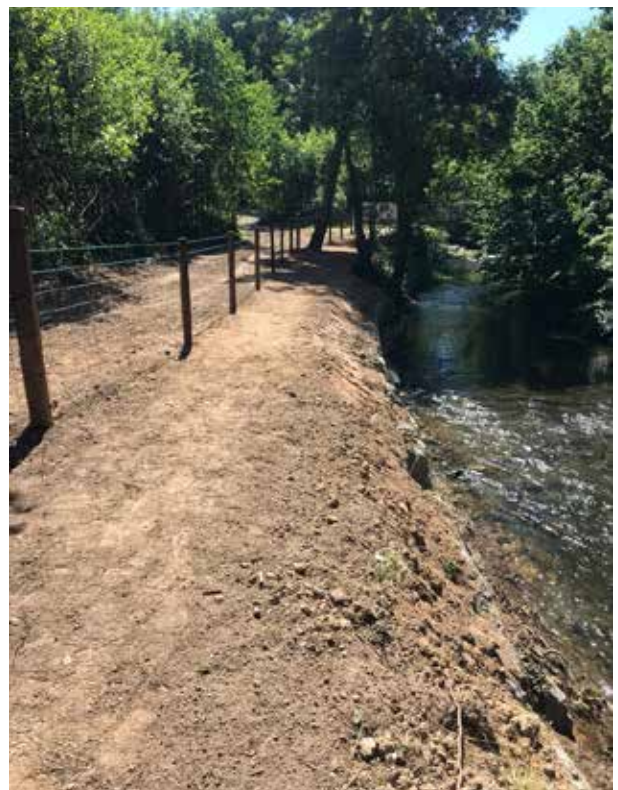
Newly erected fencing long the banks of the Ballyfinboy River.
