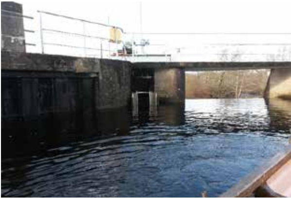
The new stainless-steel frame and fish counter on the upper side of Gweedore Weir.
