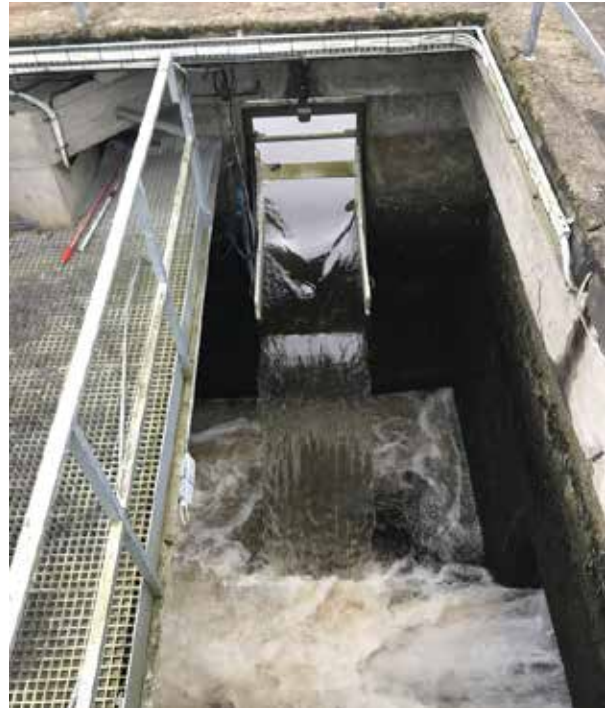
Water spilling into the upper entry point of the Leixlip station Borland fish lock, during the 2022 salmon smolt and elver generation protocol.
