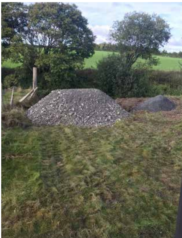
Stone fill being used for the creation of a livestock drinking area.
