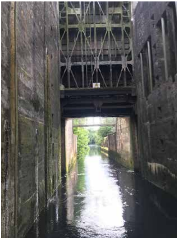
A view from the innermost section of the Ardnacrusha navigation lock.
