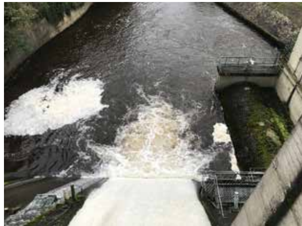
Water spillage through the 'trash flap' gate at Leixlip station as part of the 2022 smolt generation protocol.
