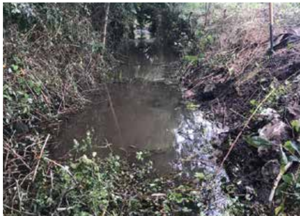
Clearance of a heavily tunnelled stream on the River Hind system.
