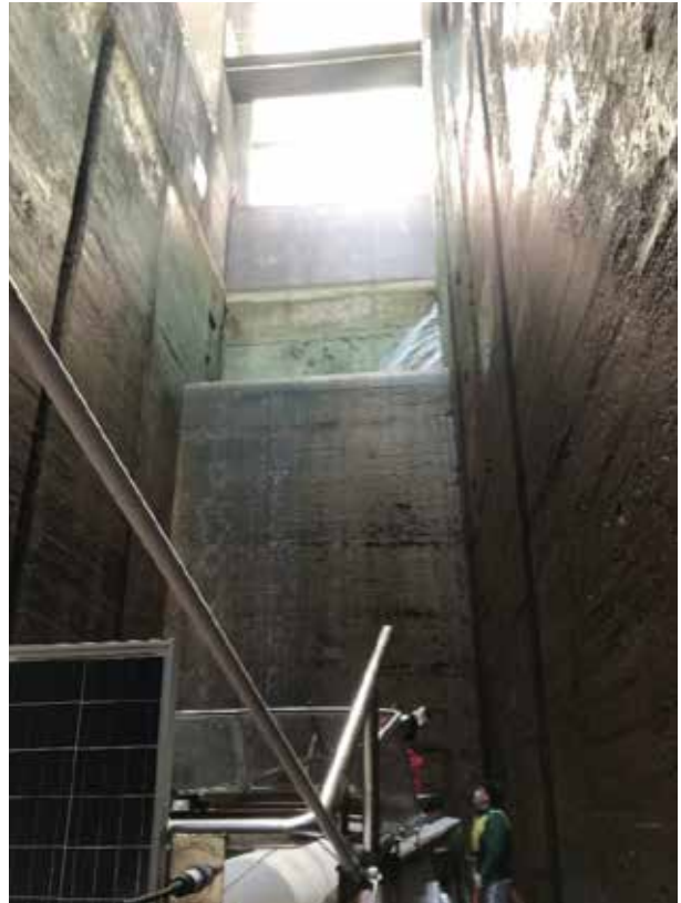
A view of the Ardnacrusha navigation lock looking upstream.
