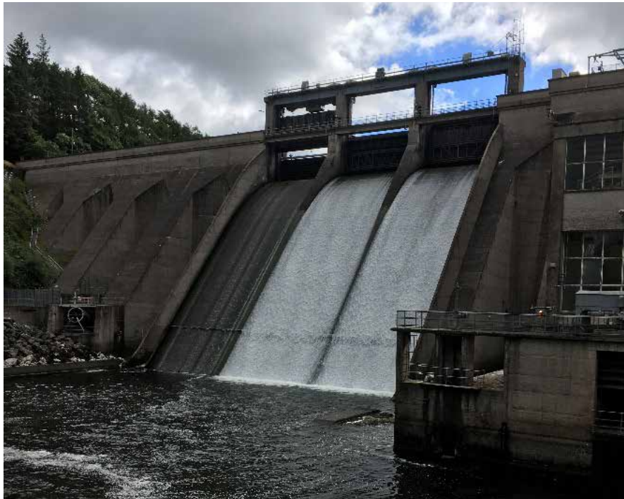
Iniscarra station showing the summer spillage of oxygenated water which is the River Lee statutory minimum flow.
