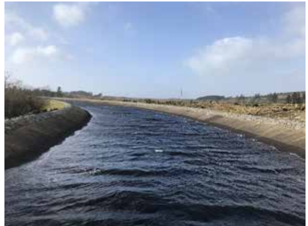
A view of the Clady station headrace canal
