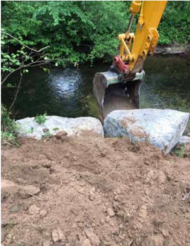
A short section of rock armour being built on the Ballyfinboy River.
