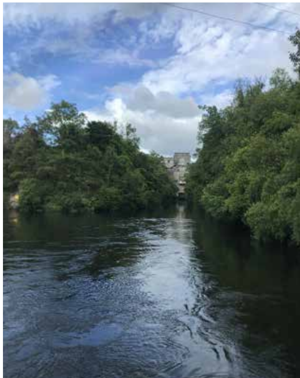
A view of the lower section of the navigation lock in Ardnacrusha station.
