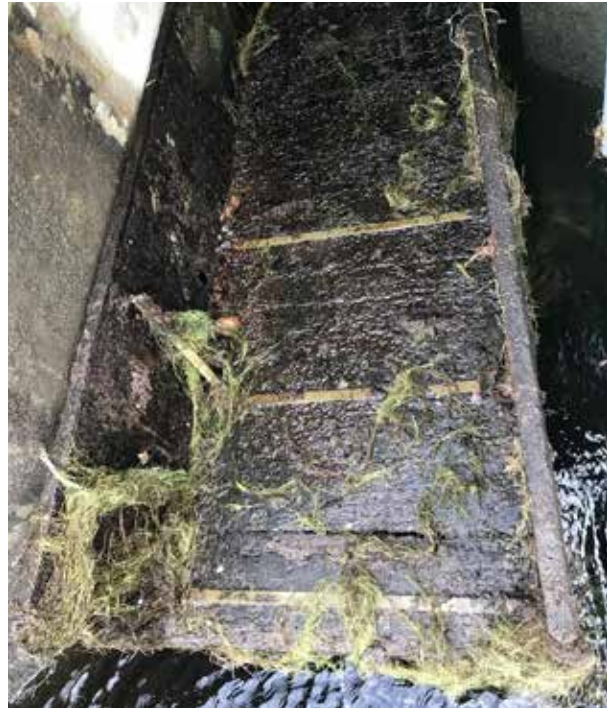
The old fish counter chute which holds the fish counter scanning unit at the upper exit point of the Gweedore Weir fish lock.
