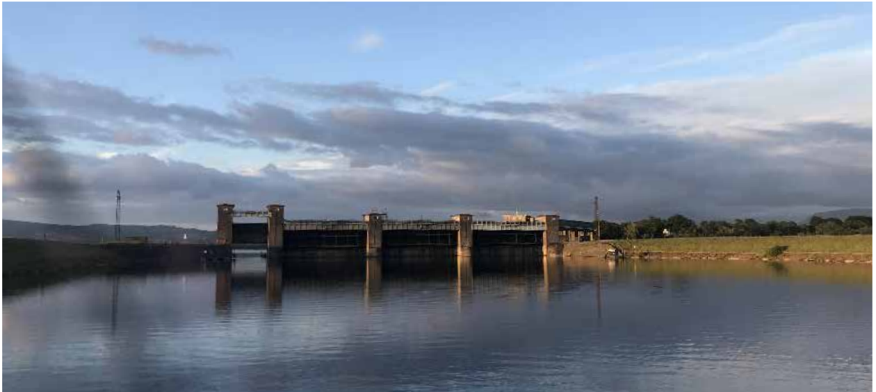
The regulating gates at the entry point to the Ardnacrusha headrace canal.
