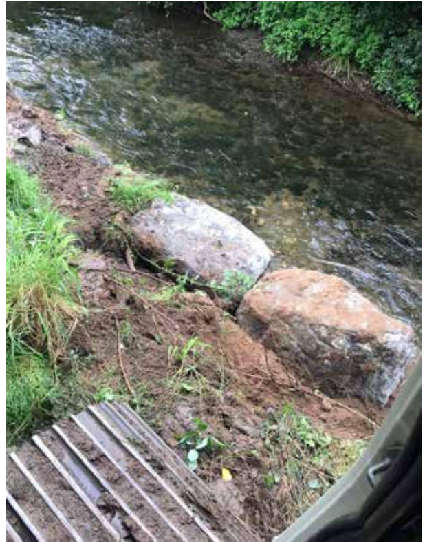
A short section of rock armour being built on the Ballyfinboy River.
