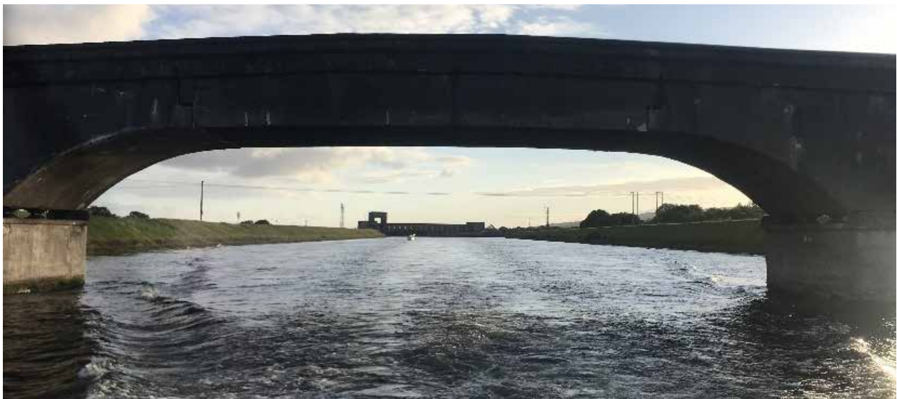
An upstream view of Ardnacrusha station and headrace canal.
