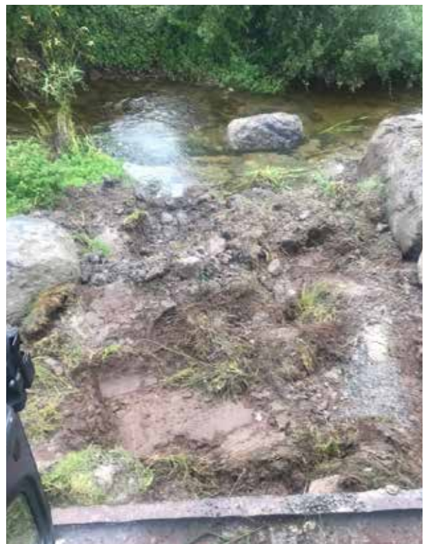
A random boulder being placed into the Ballyfinboy River.
