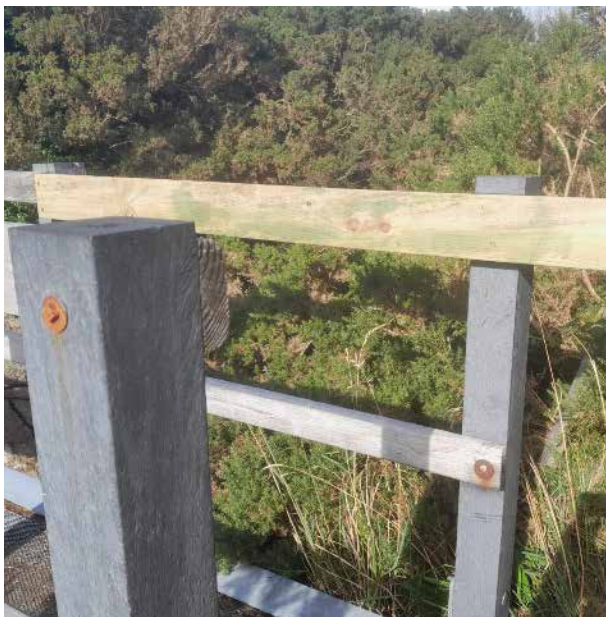
Replacement of a handrail on the Iron Bridge Clady
