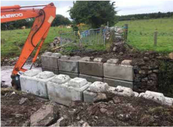
The provision of a cattle crossing point over a tributary of the River Hind.
