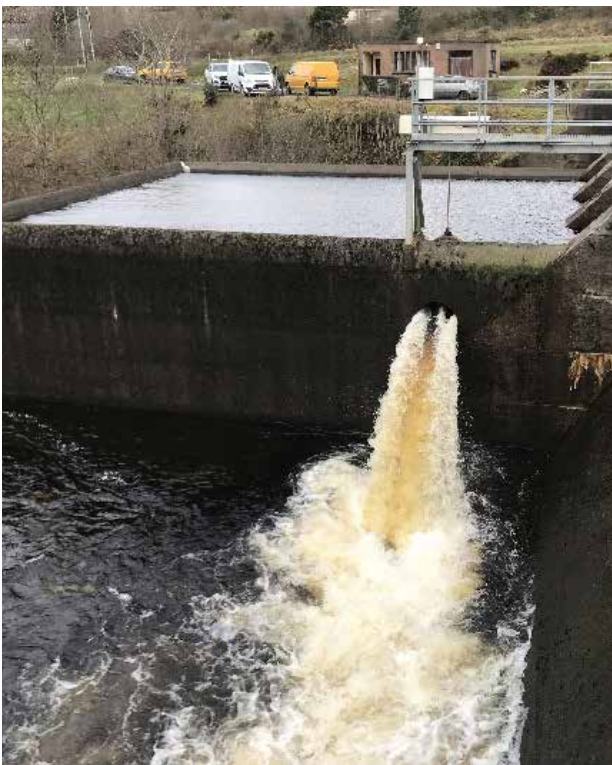
A summer freshet being discharged through Gweedore Weir on the Clady River.
