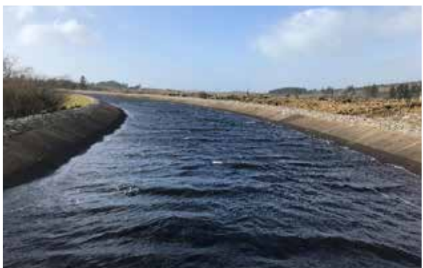
Views of sections of the Clady headrace canal which used to divert water from the Clady River for hydroelectric generation.
