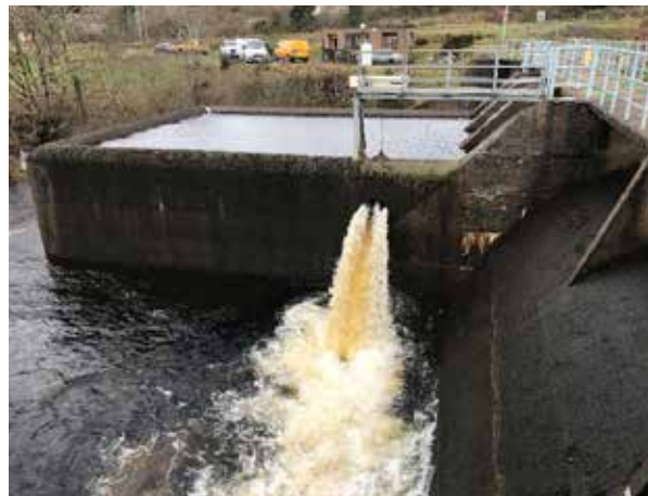
A view of the freshet discharge valve located at Gweedore Regulating Weir.
