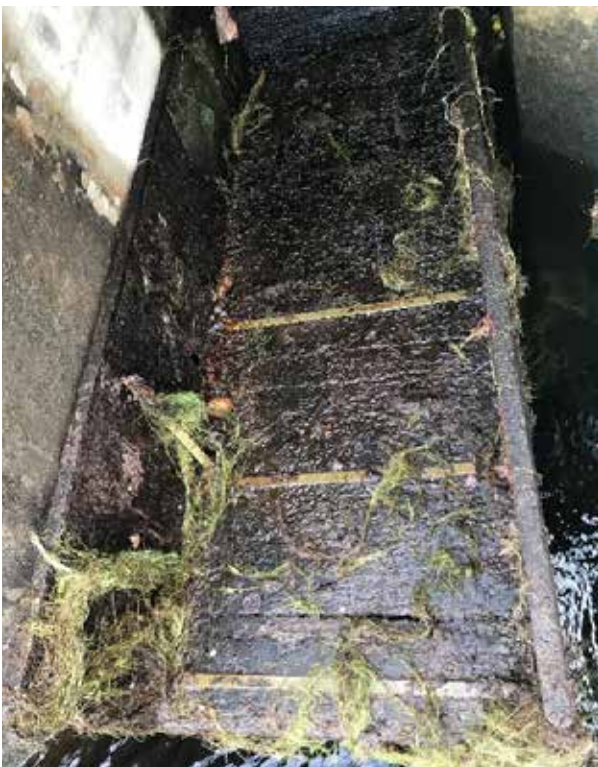
The old wooden cradle which previously held the scanning units which generated data on fish movements and numbers at Gweedore Regulating Weir. This will be replaced with a new stainless steel cradle in 2022
