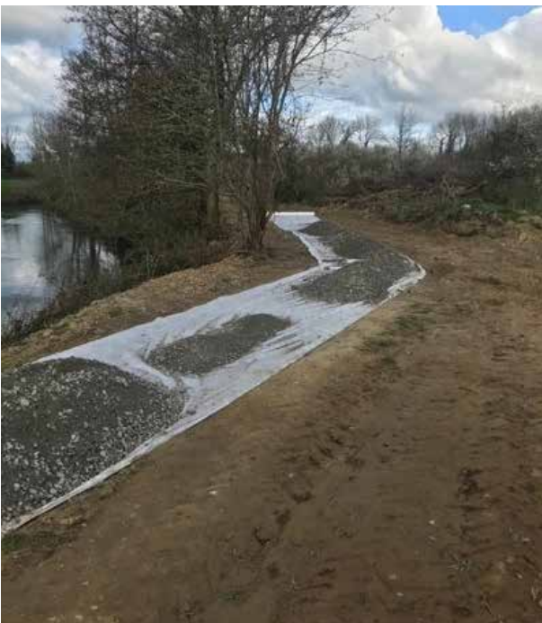
A new footpath being constructed along the banks of the Nenagh River.
