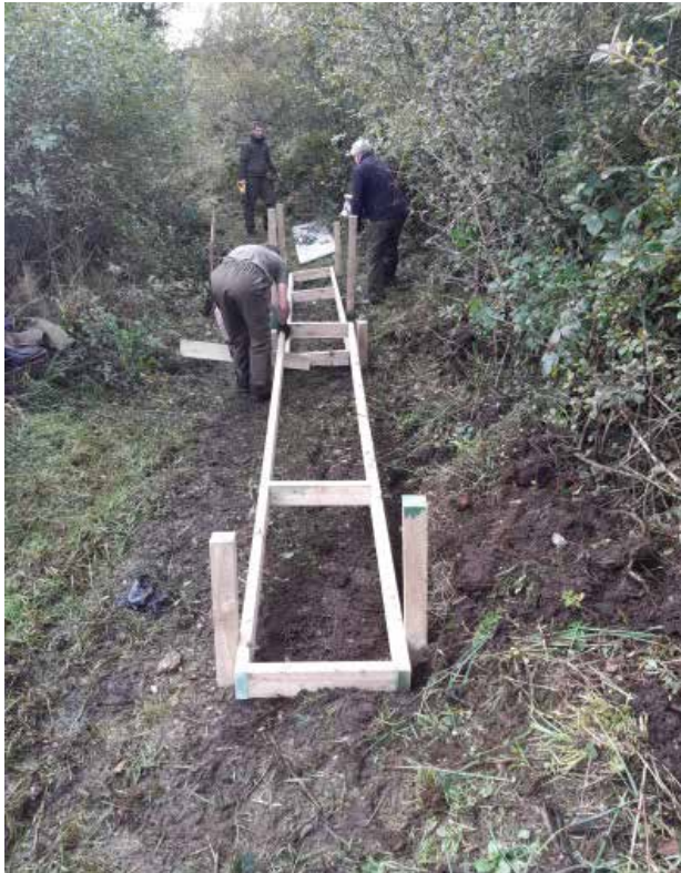
A new walkway being constructed on the Crollly River.
