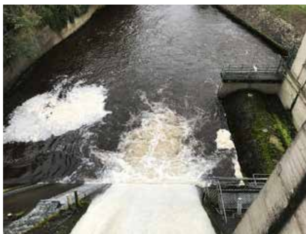
Photographs of flood water being discharged through the spillway gates at Leixlip station on the River Liffey.
