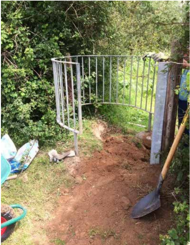
ESB staff repairing gates alongside the Mulkear River.
