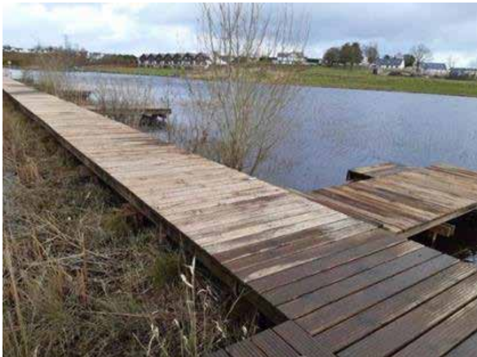
Repairs and maintenance to the angling stands at the mudflats, Carrick-on-Shannon.
