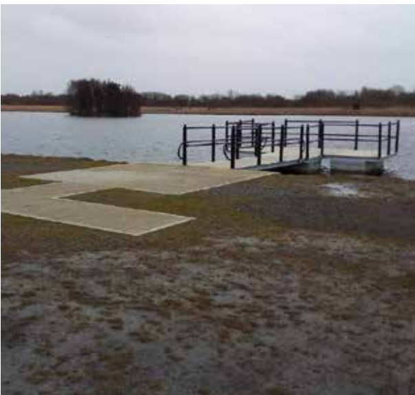
Views of a floating-pontoon type wheelchair accessible structure erected on Cloghan Lake.
