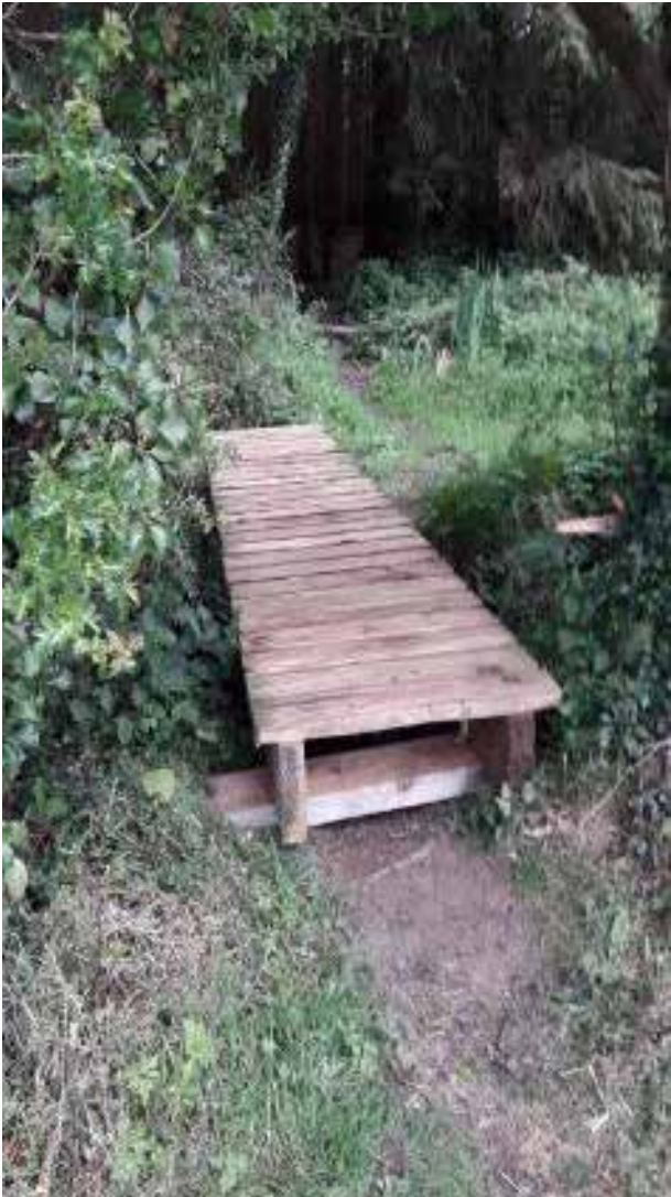
Temporary footbridge at Reddan's Quay, Tuamgraney.
