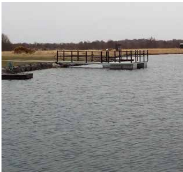
Views of a floating-pontoon type wheelchair accessible structure erected on Cloghan Lake.
