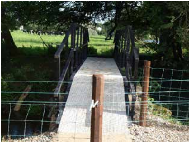
The new footbridge over 'Conway's Canal' in Castleconnell.
