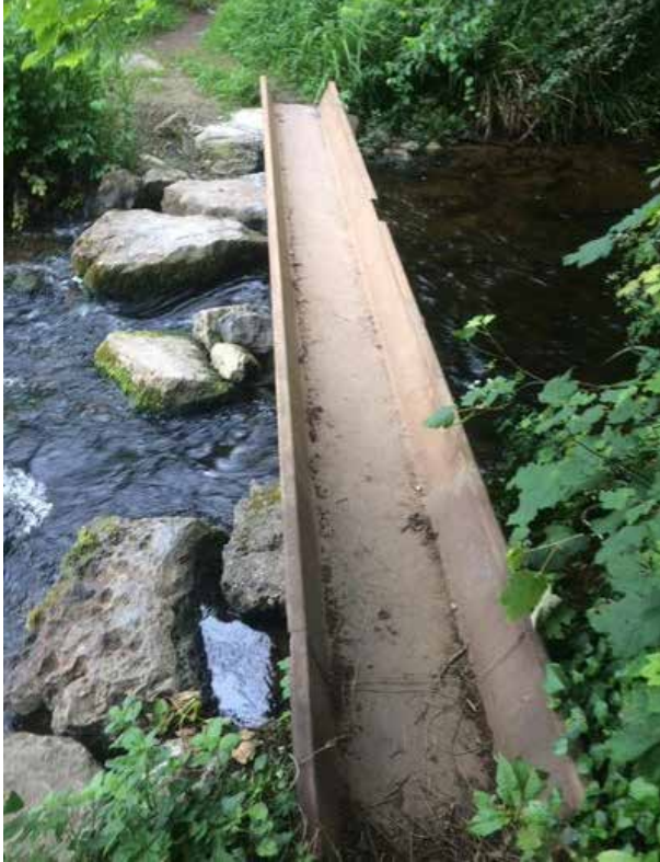
An old footbridge structure and a barrier to fish migration identified on the Newport River (a tributary of the Mulkear), Co. Tipperary.
