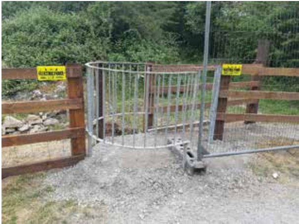
Views of the swing-gate and fencing beside 'Conway's Canal' in Castleconnell.
