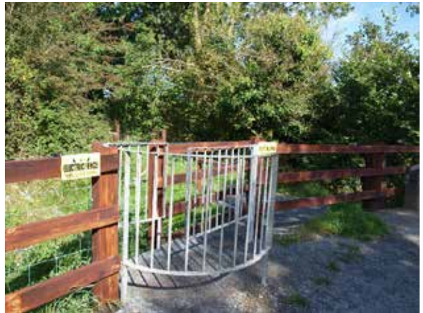
A new swing gate and fenced area near adjacent to 'Conway's canal'.
