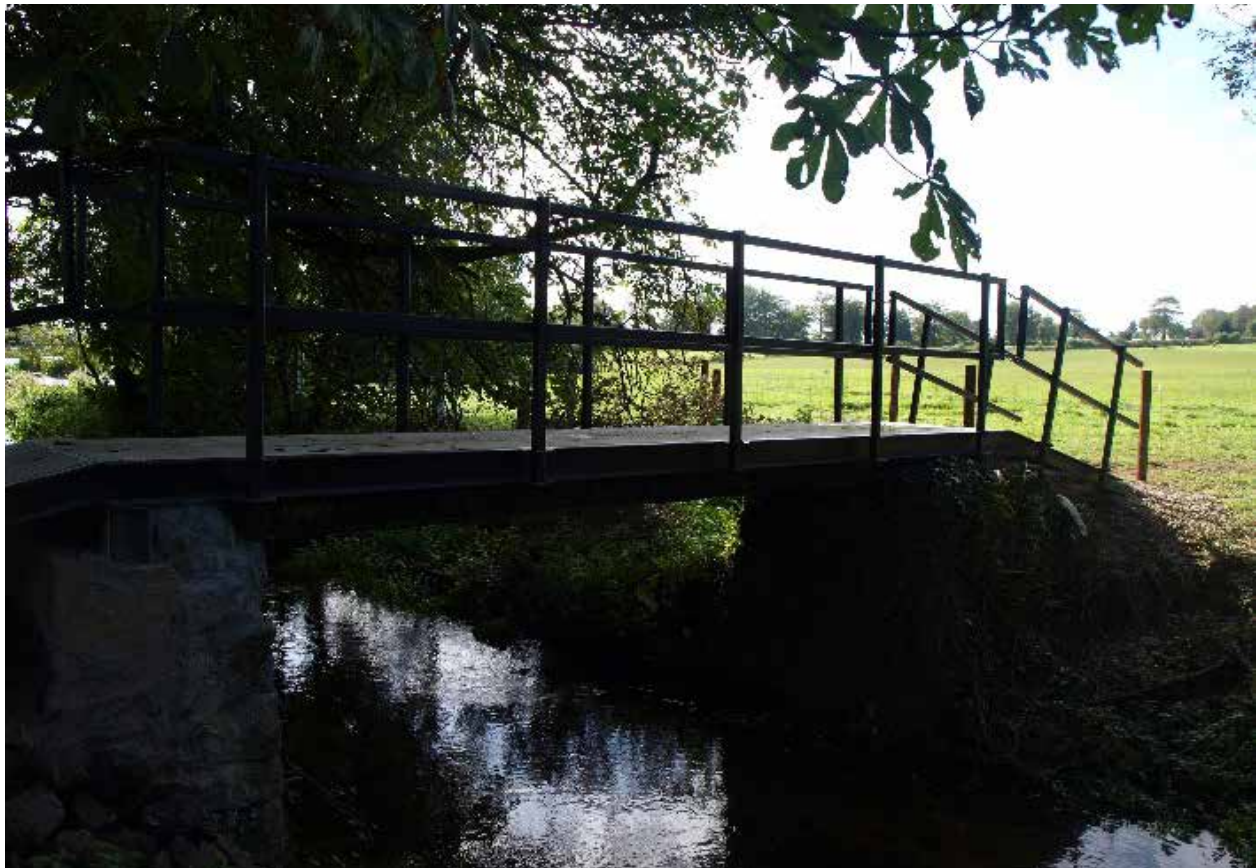
The new footbridge over 'Conway's Canal' in Castleconnell.
