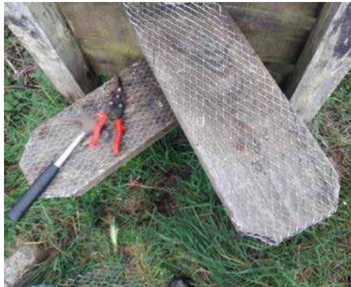
Repairs to stiles on the River Feale, County Kerry.
