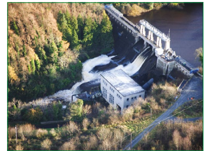
The 86 MW hydroelectric power station on the Shannon at Ardnacrusha
