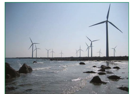
The 12 MW wind farm at Carnsore Point with its 14 turbines
