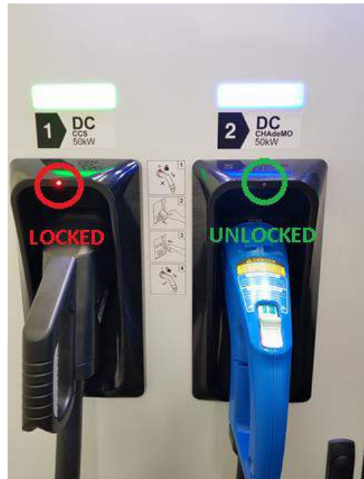
Figure 7. CHAdeMO Connector unlocked
