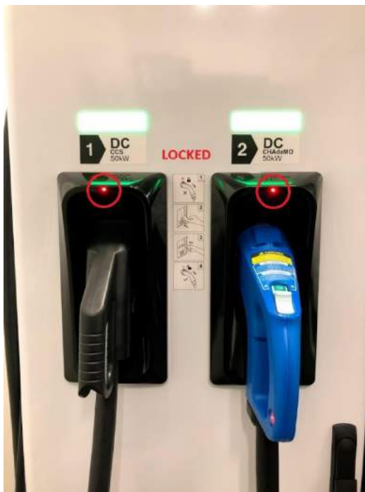
Figure 8. Connectors locked
