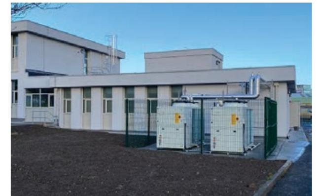
Energy efficient heat pumps provide water and space heating to the building.
