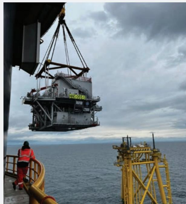
The first of the two offshore substations being lifted onto its foundation jacket at Neart Na Gaoithe offshore wind
