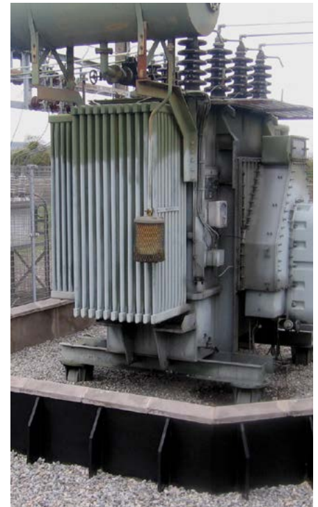
A retrofit HDPE bund
