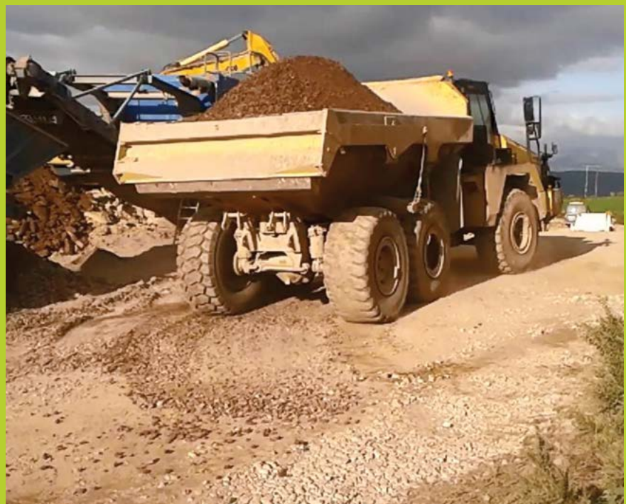
Materials management at Woodhouse wind farm construction site in Co. Waterford.
