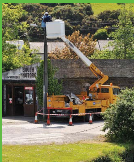
Work at one of the Single-Phase Transformers.
