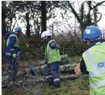
ESB Networks staff during work in Killarney.
