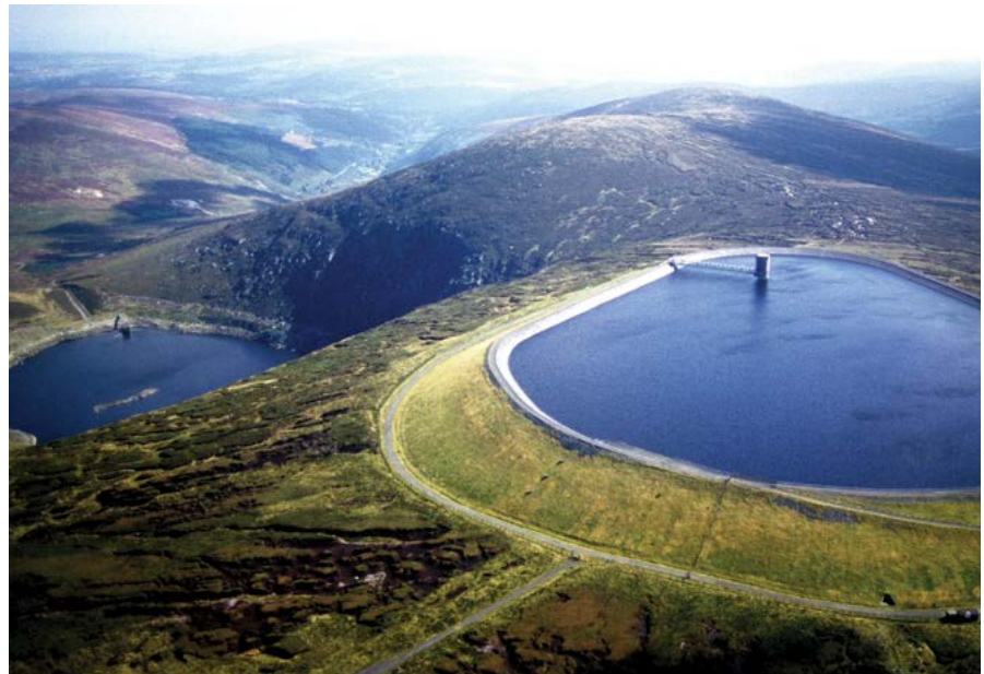
Turlough Hill Pumped Storage Station in Co Wicklow.
