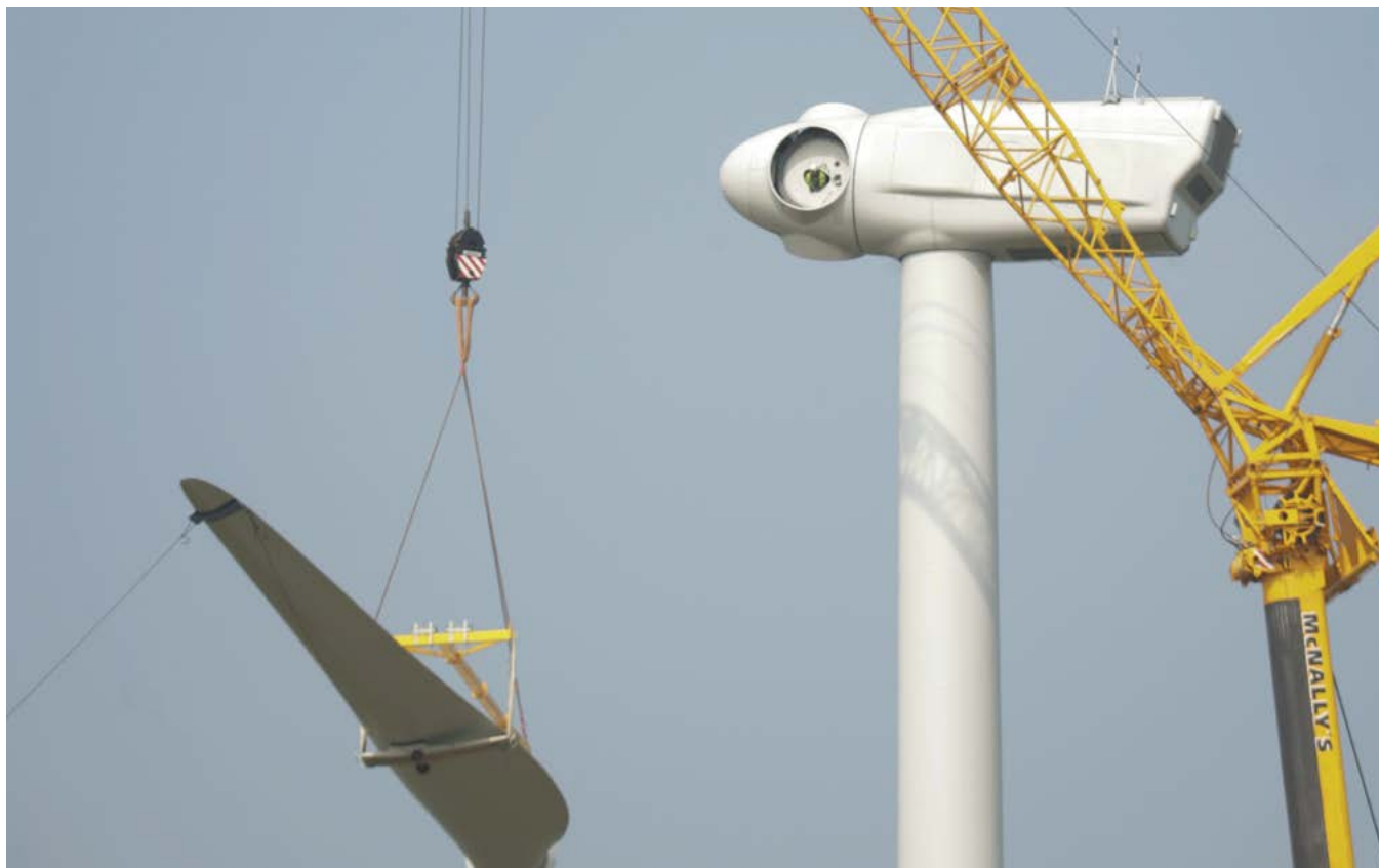
Crane erecting a turbine blade during wind farm construction
