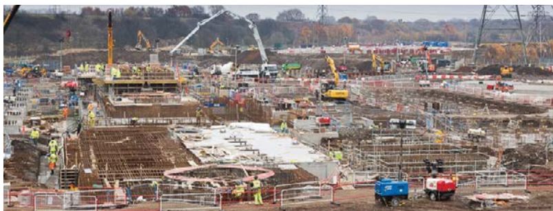
Power Train Foundation, Unit 1 steelwork.
