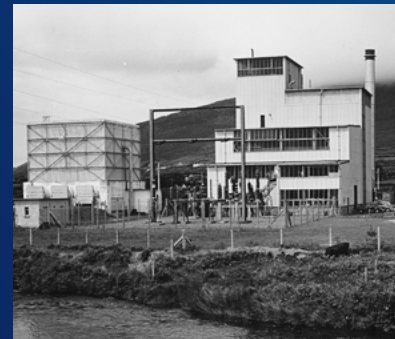
← The peat-fired power stations built by ESB – such as this one in Cahirciveen – in the 1950s and 60s delivered economic benefits and employment to rural areas.
