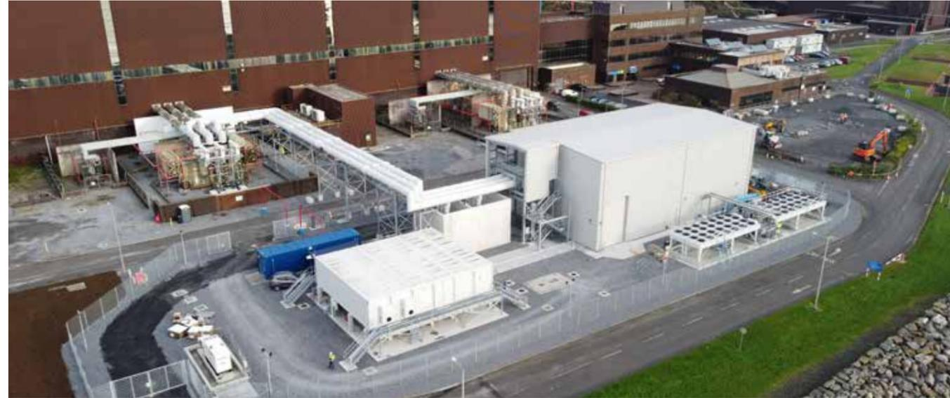
The Synchronous condenser and flywheel at Moneypoint, will enable the connection of greater levels of intermittent renewables to the electricity grid by providing improved voltage regulation.
